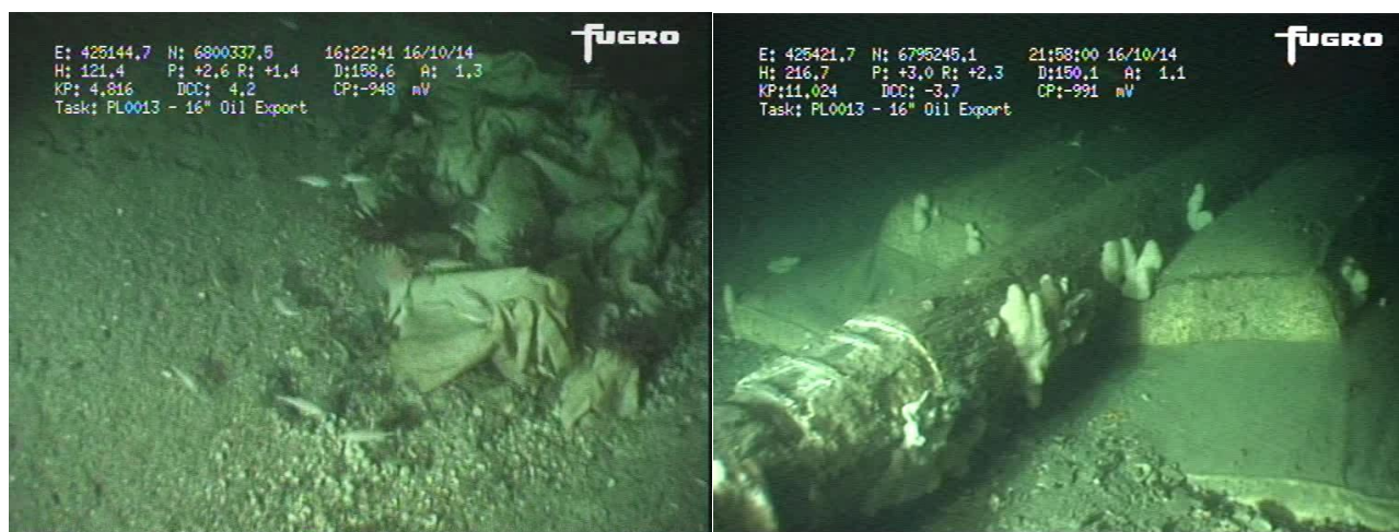
Figure 3.5.1: Examples of grout mattresses used for remediation (2014)
