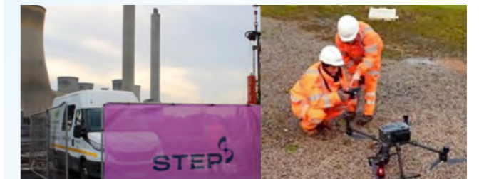
Borehole drilling and drone capture to characterise the site
