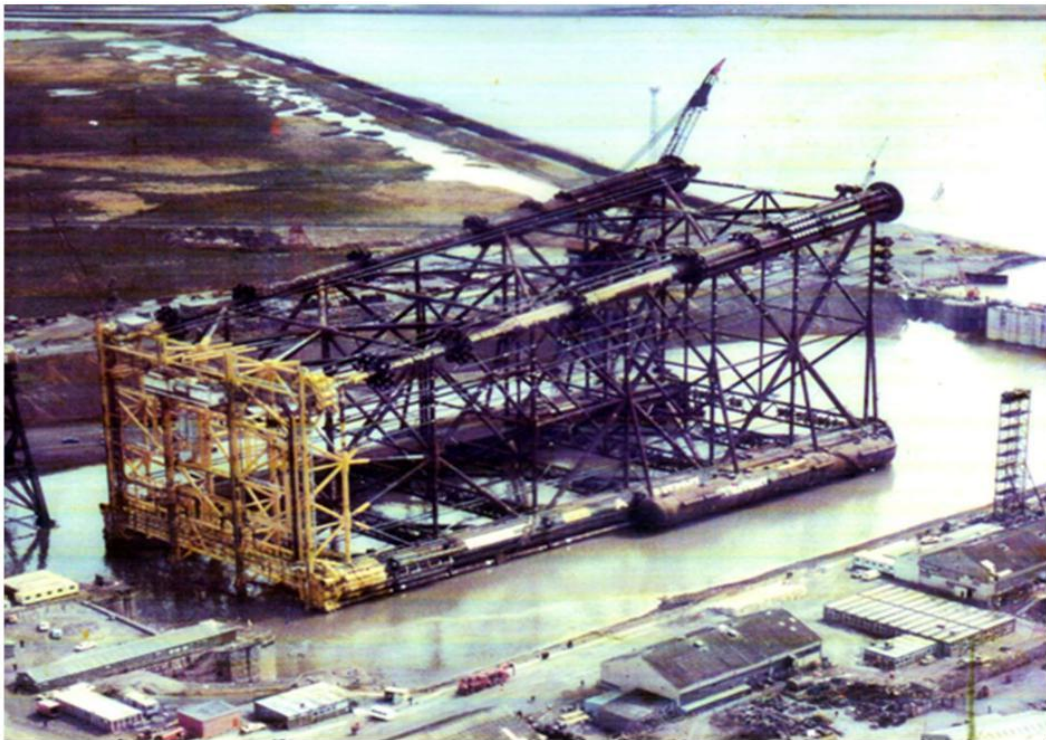
Figure 2.1.6: Thistle jacket fabricated at Greythorpe Dry Dock, Middlesbrough
