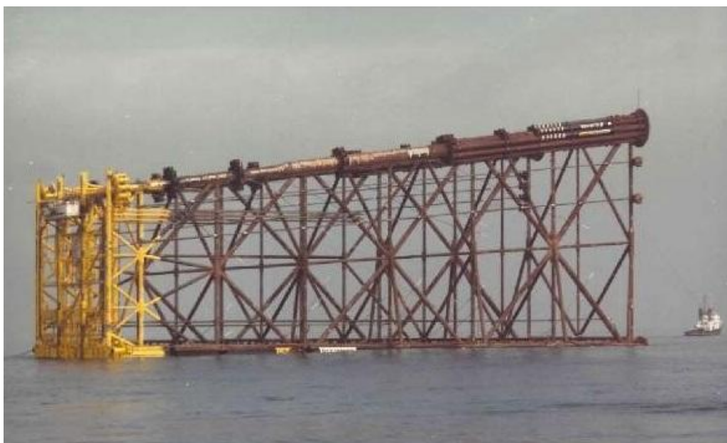
Figure 2.1.7: Thistle jacket immediately prior to upending
