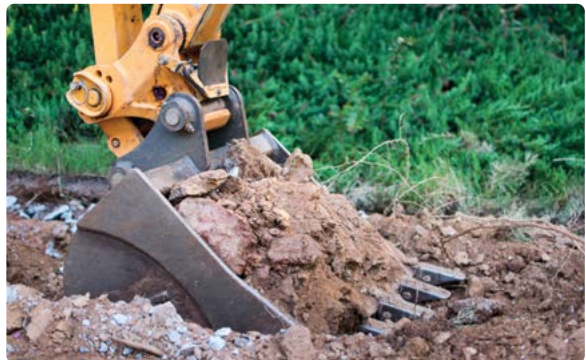
Pit or trench dug to investigate soil conditions from the surface and to obtain samples. Image: Hs2 Ltd.
