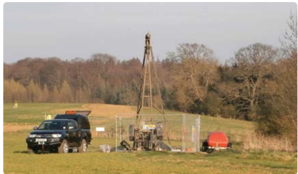
Cable percussion borehole. Image courtesy of CH2M.
