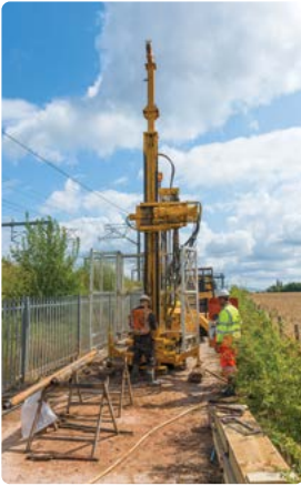
Drilling of a small borehole via a rotary core rig. Image: HS2 Ltd.
