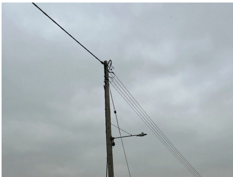
Figure 10: Photo showing bundled aerial conductor on the left of the pole and unbundled 4-wire construction to the right of the pole
