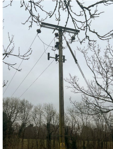
Figure 6: Examples of 6.6 kV three-phase overhead lines
