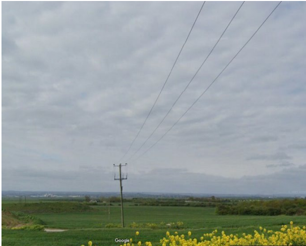
Figure 6: Examples of 6.6 kV three-phase overhead lines
