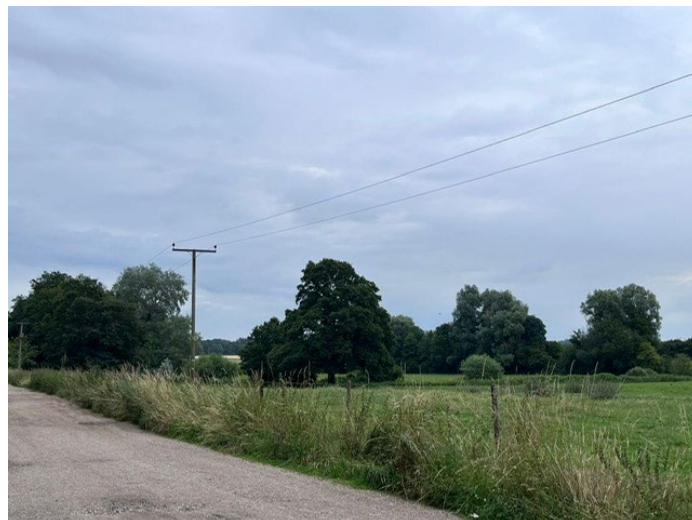
Figure 7: An 11 kV single-phase overhead line
