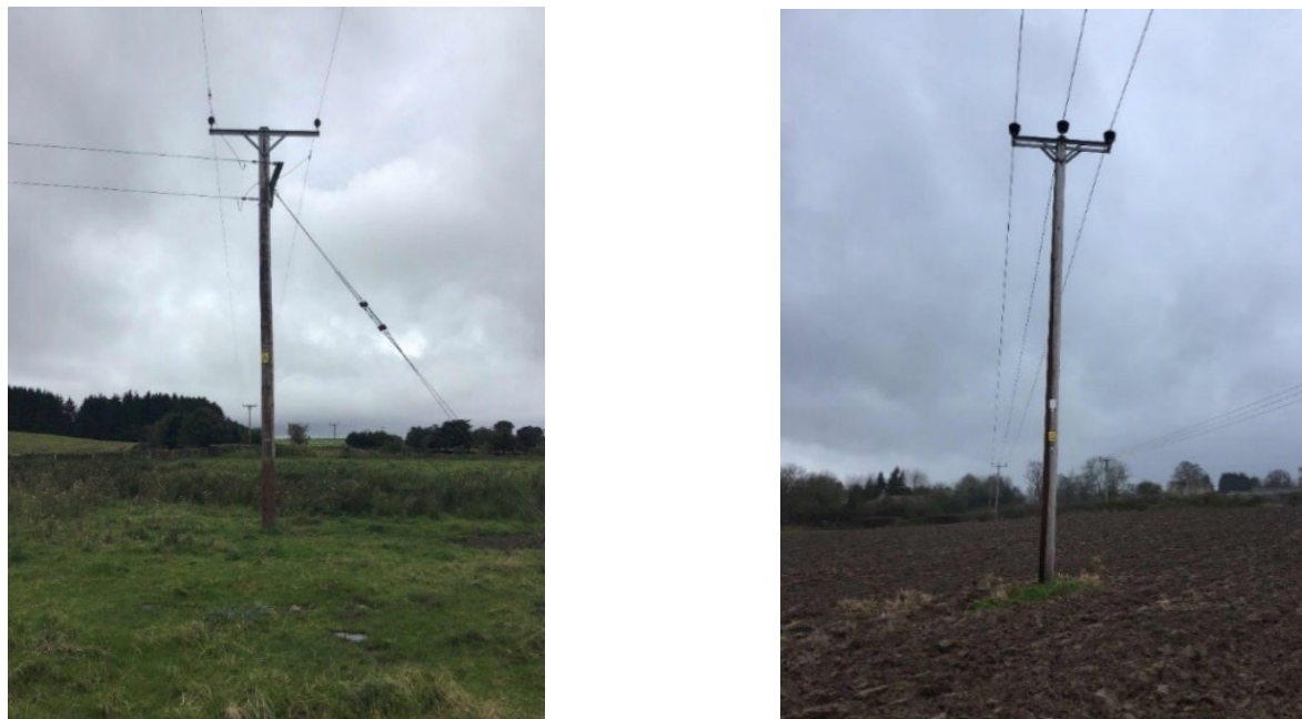
Figure 8: (Left) A 33 kV two-phase overhead line (Right) A 20 kV three-phase overhead line
