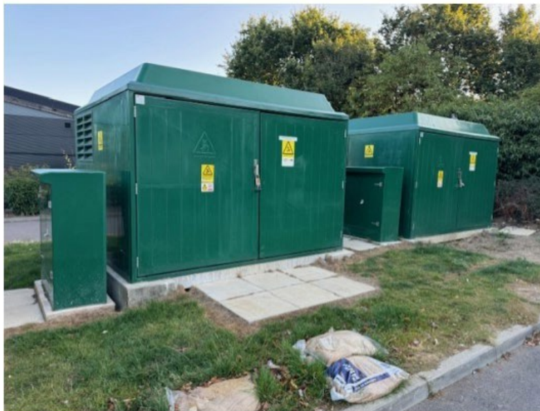
Figure 2: Two substations installed next to each other to provide capacity for electric vehicle charge point supply at a motorway service station. 17
