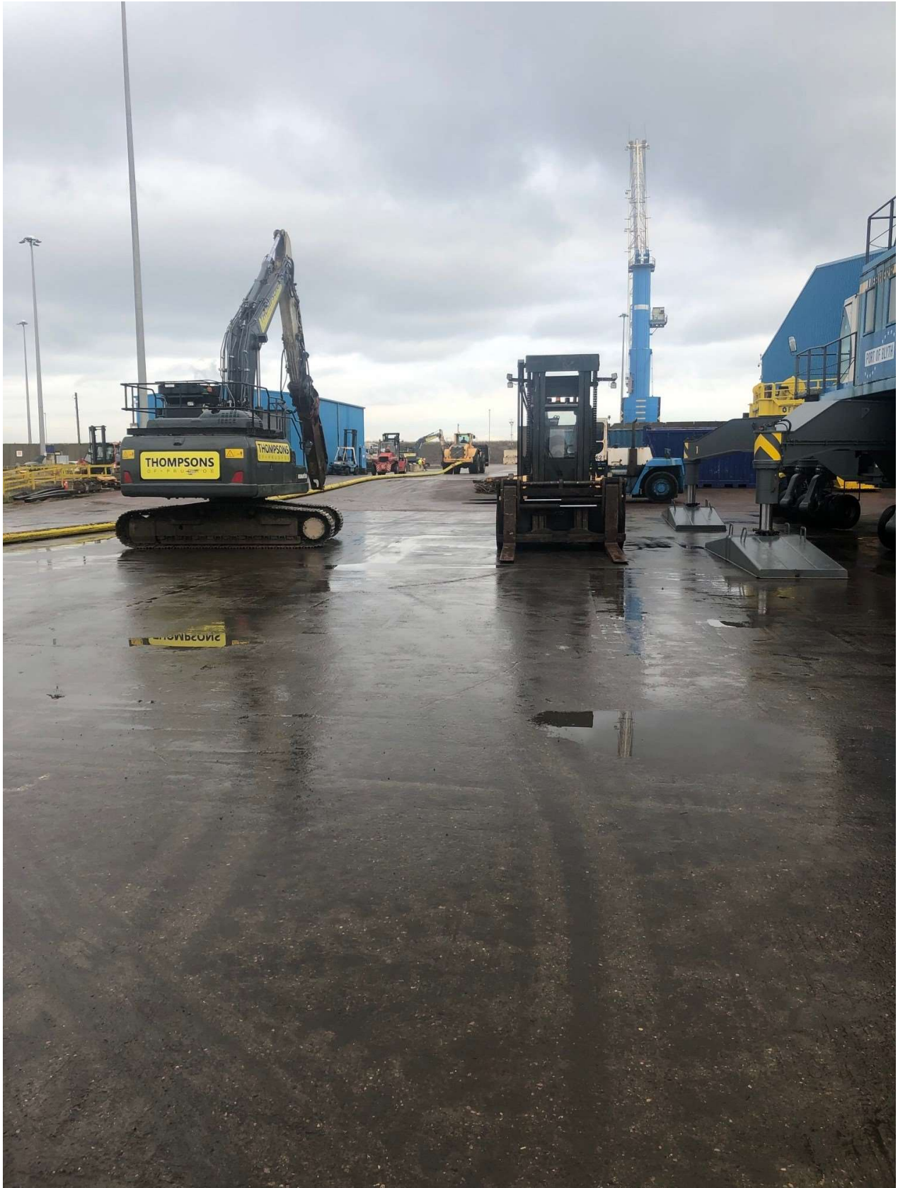
Figure 8.9.2: Riser offloading, quayside set up II
