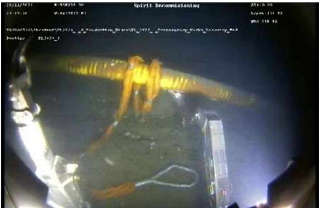
Figure 8.3.2: Typical rigging arrangement for product recovery
