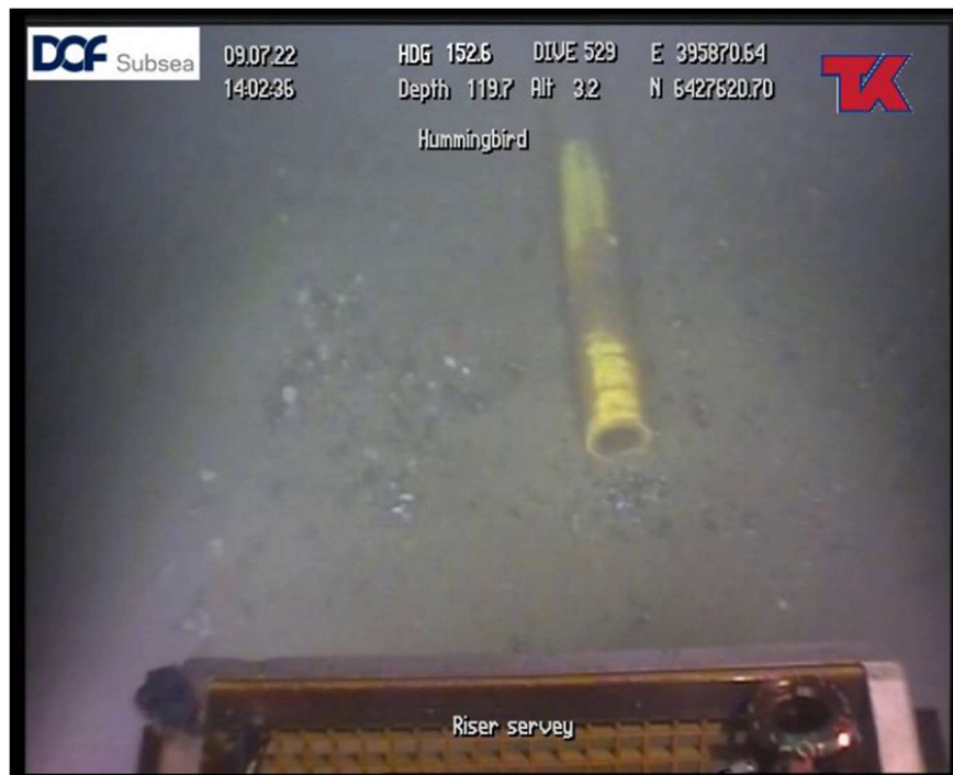
Figure 2: Production riser cut end
