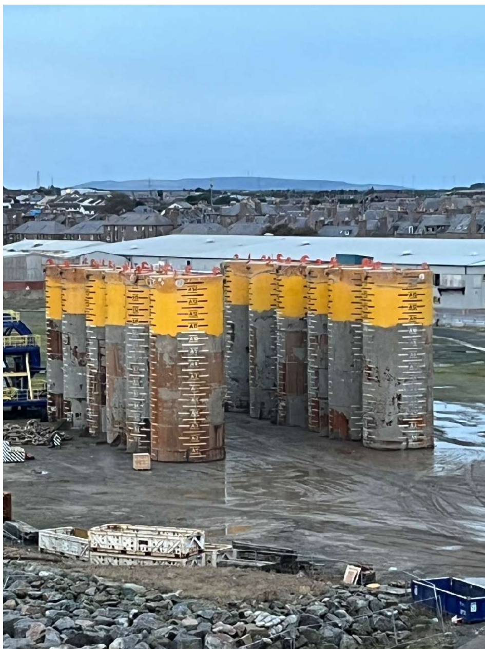
Figure 8.1.3: Sevan Hummingbird FPSO 12x suction anchors
