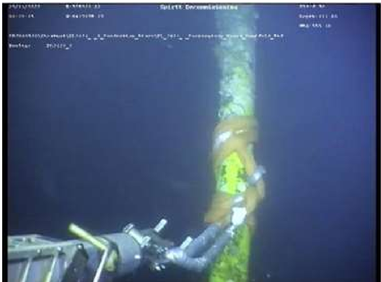
Figure 8.3.3: Typical hold-down rigging arrangement before product recovery
