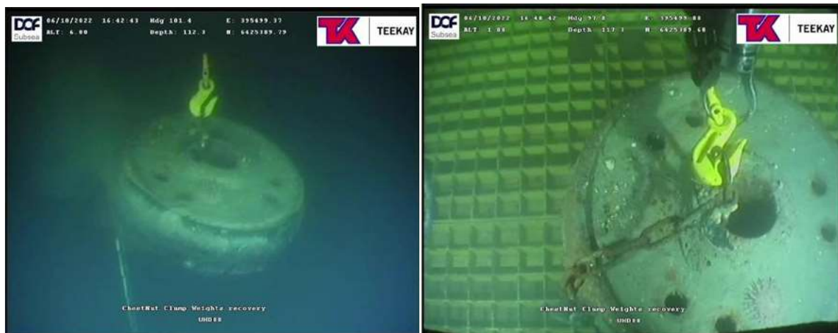
Figure 8.2.1: Wave rider buoy clump weight #3 being recovered
