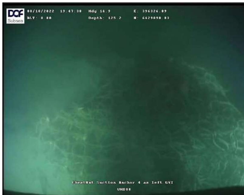
Figure 8.3.1: Suction Anchor 4 – Fishing Net
