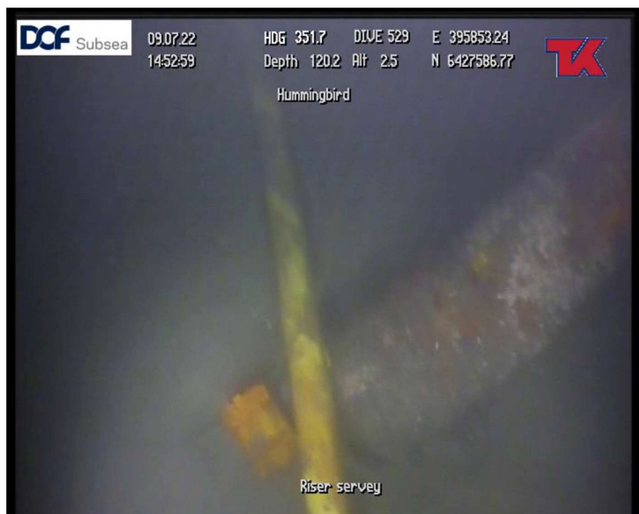
Figure 8: Water injection riser cut end
