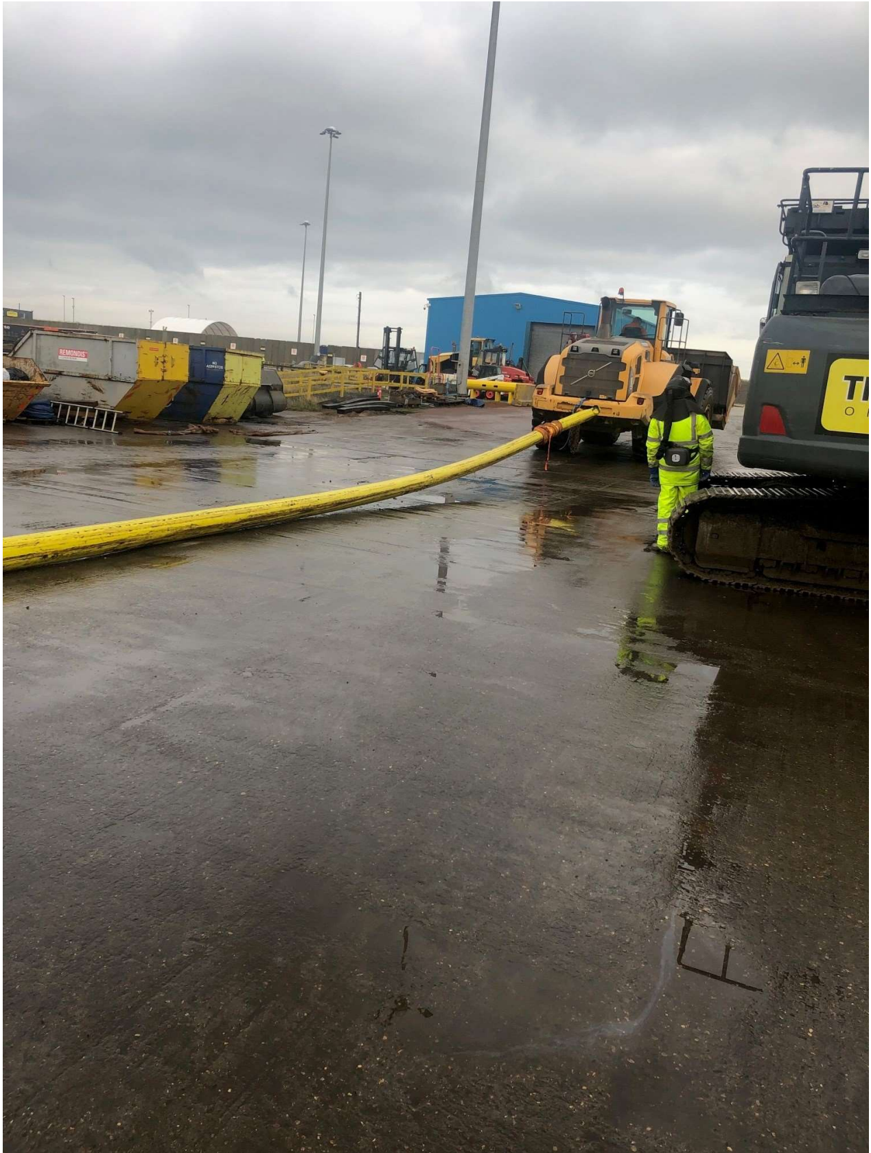
Figure 8.9.3: Riser offloading, towing tractor
