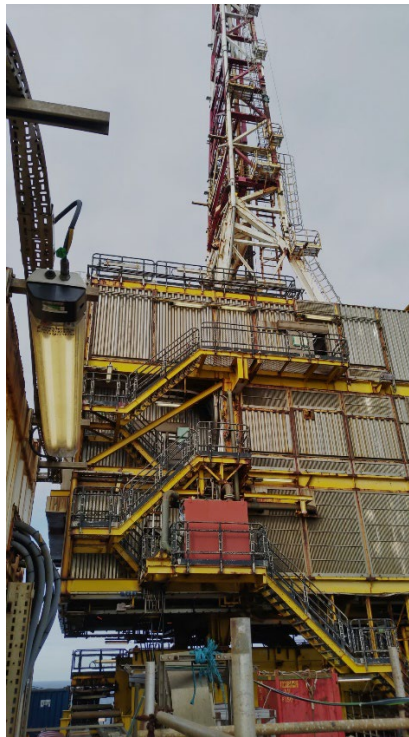
Figure 2.1: Gannet A drilling substructure with Mast
