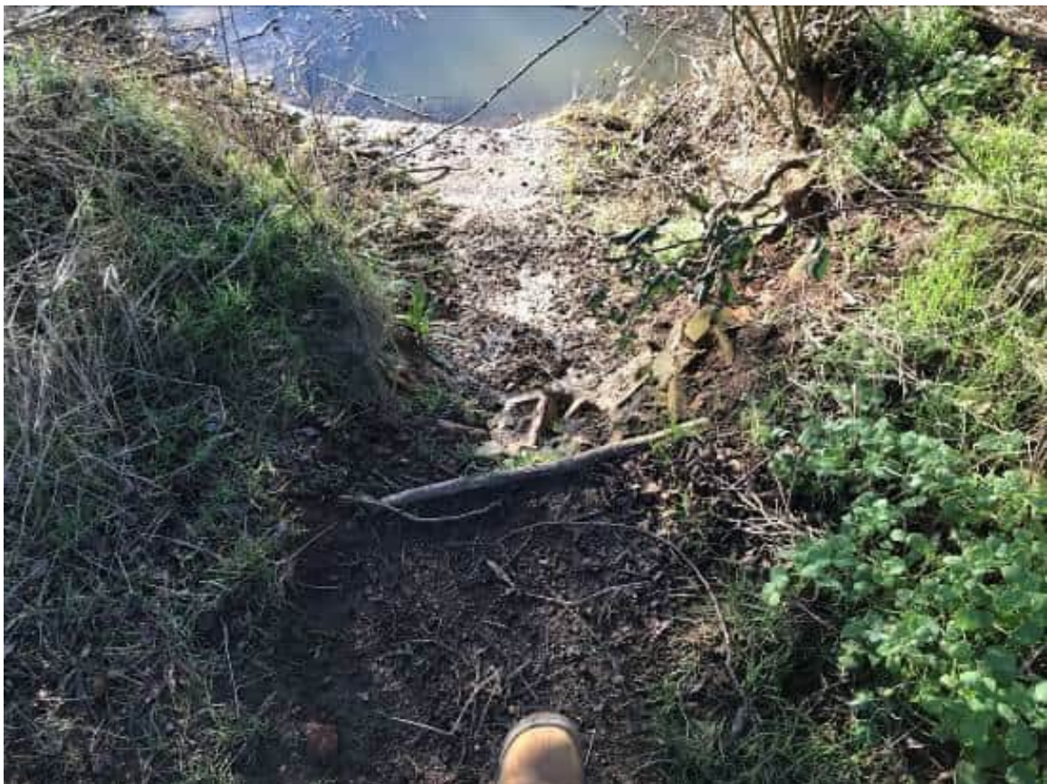
View of erosion along upstream face
