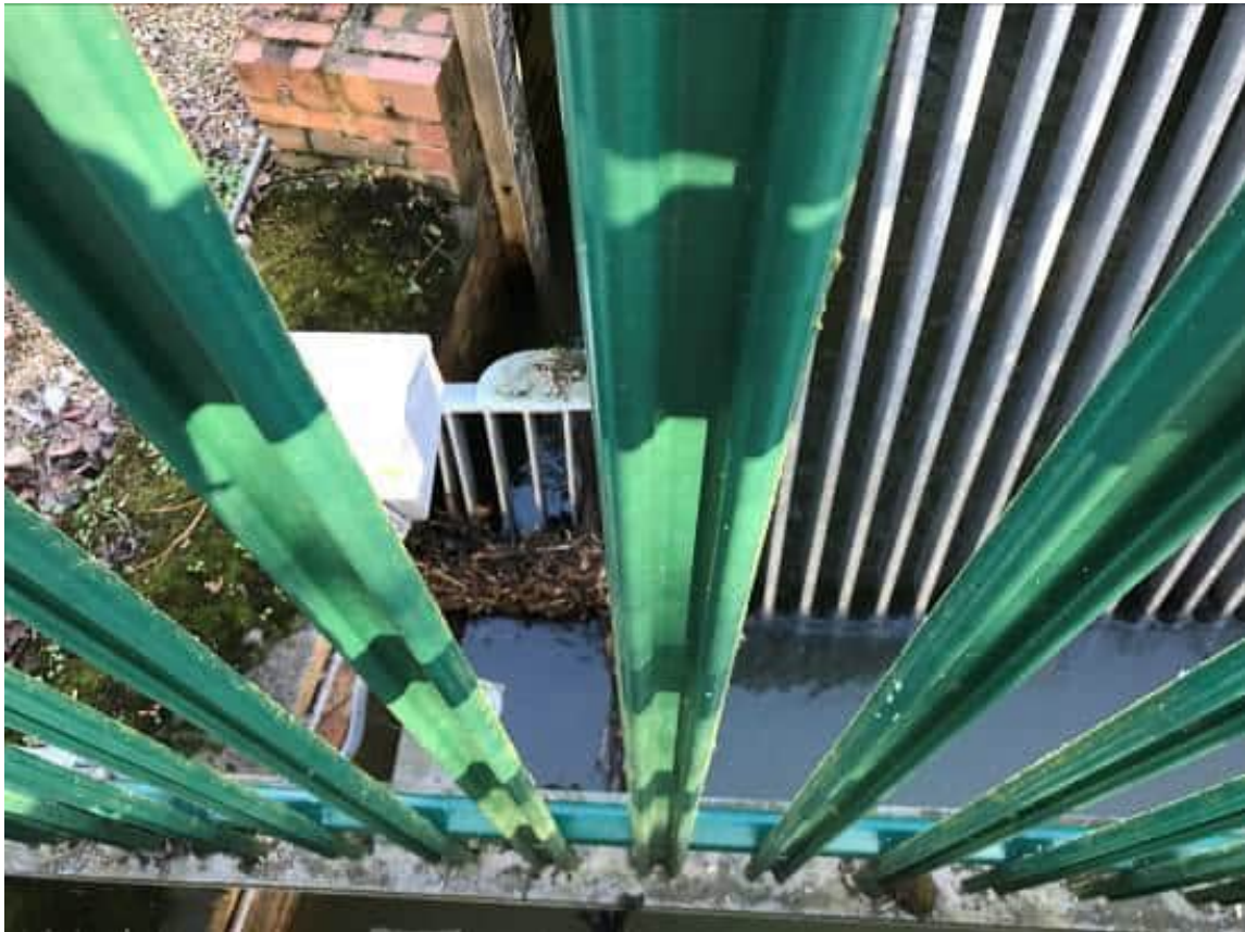
View of gauge board and low level debris screen
