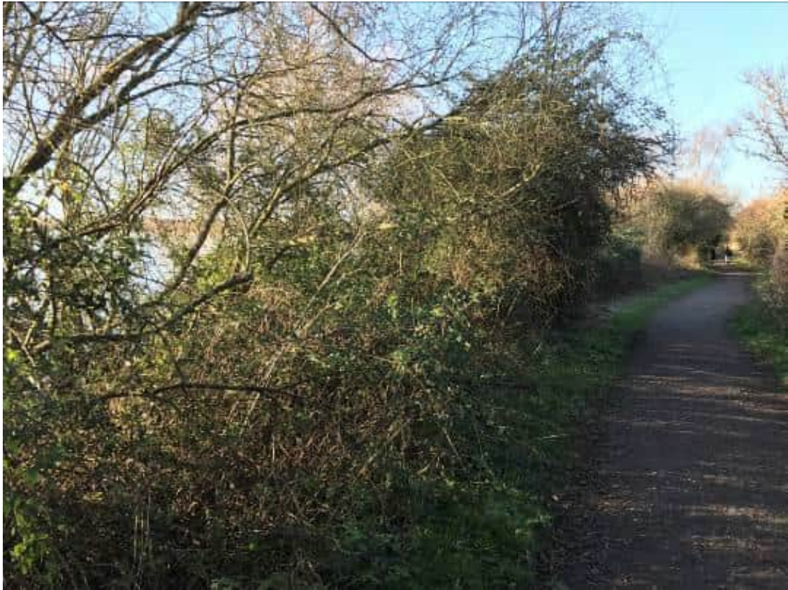
Vegetation along upstream face of embankment
