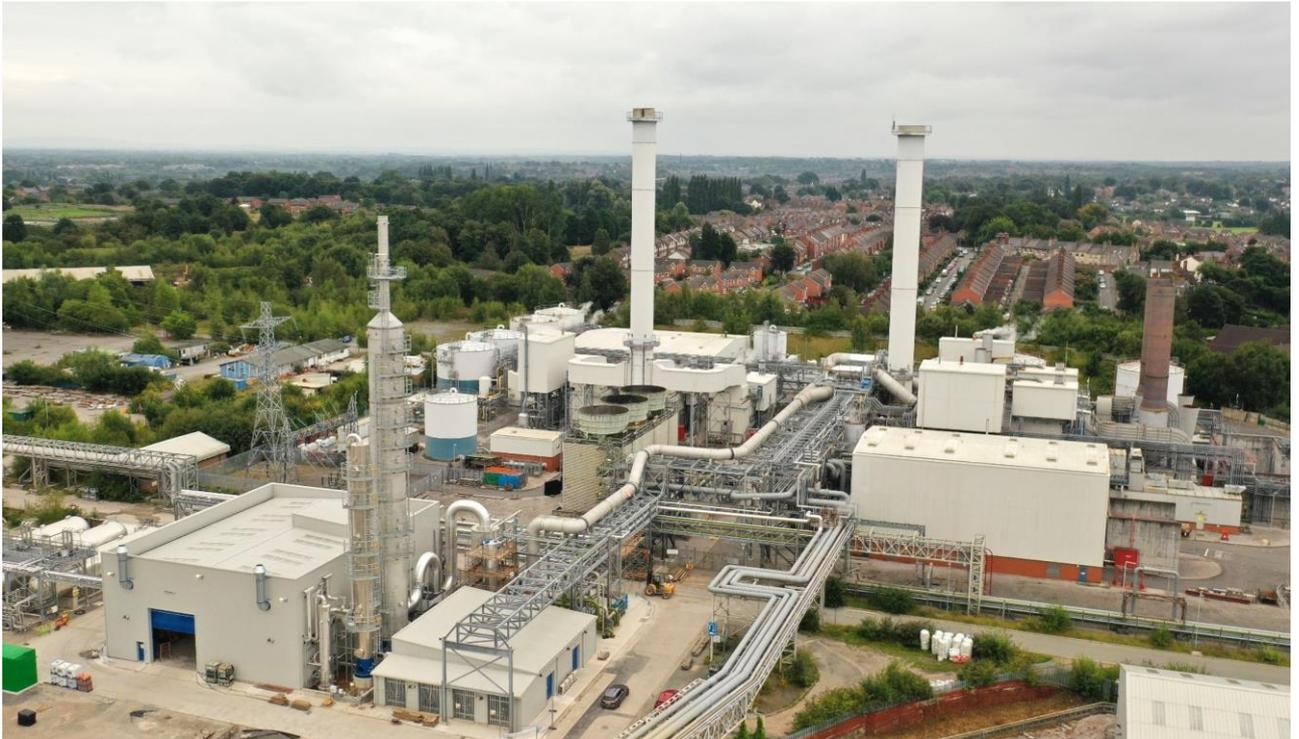
**Figure 11: Tata Chemicals Europe CHP and connected CCU plant with associated carbon dioxide absorber in foreground.**
