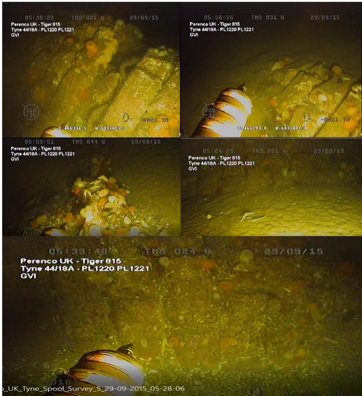
Figure 7-3: Survey images of concrete mattresses at the approach to the previous Tyne platform
