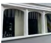
Wooden framed windows
