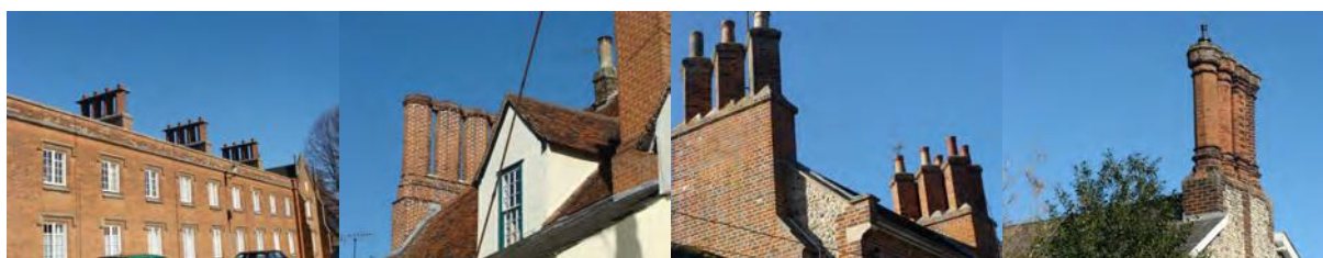
Selection of chimneys on listed buildings
