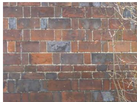
Picture 1.22 Prominent boundary wall in grounds of Elm Grove; unusual rat trap bonding
