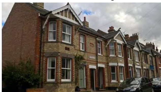
Picture 1.37 No.s 46 - 52 Fairycroft Road
