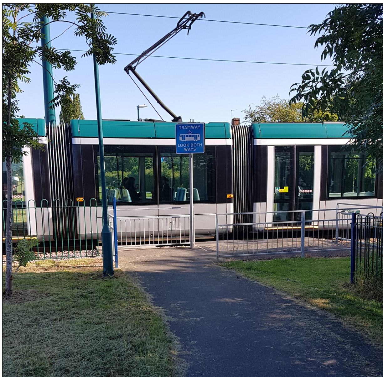
Figure 12: An example of chicane fencing on a footpath crossing on the Nottingham tram system. The tram in the picture is travelling on the closer of the two tracks from right to left.
