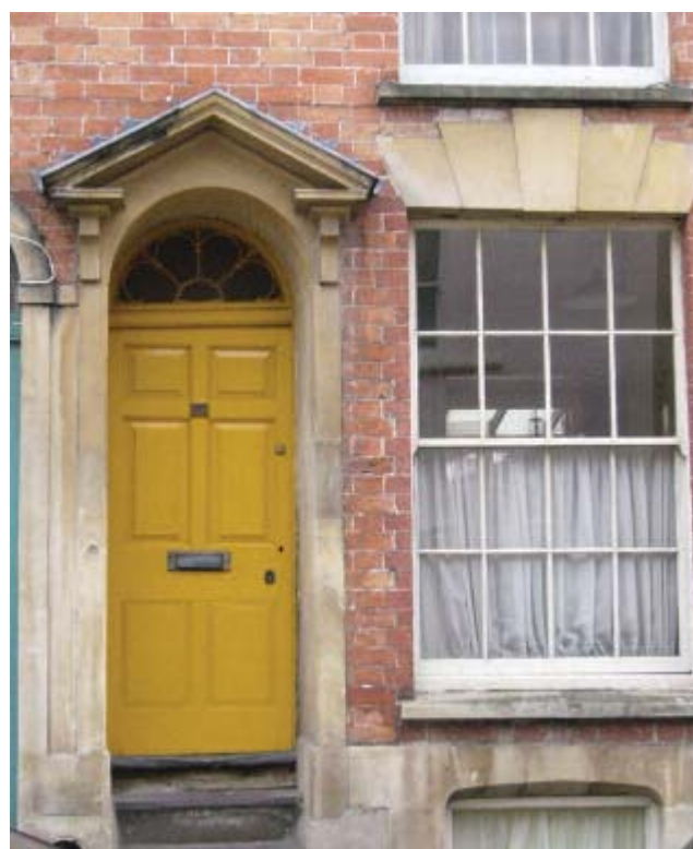
Figure 32: Limestone pedimented door surround, timber panelled door with decorative fanlight and eight-over-eight timber sash window, Picton Street
