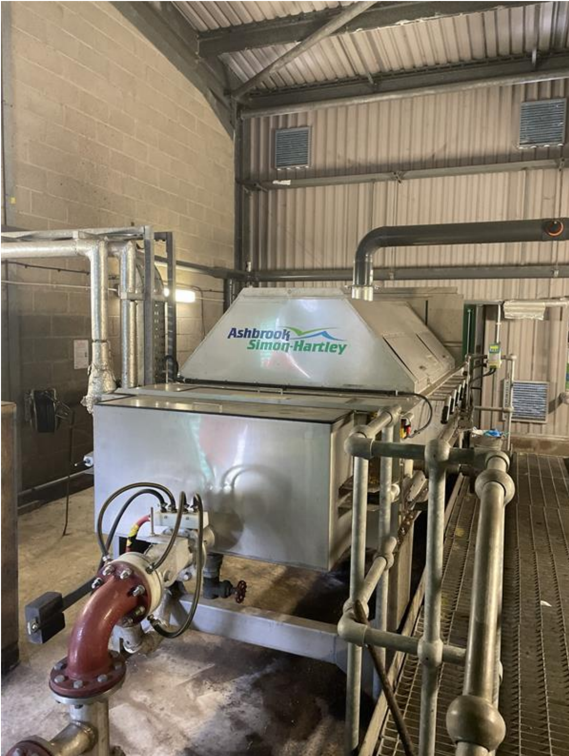
Photo 4. Gravity Belt Thickener
