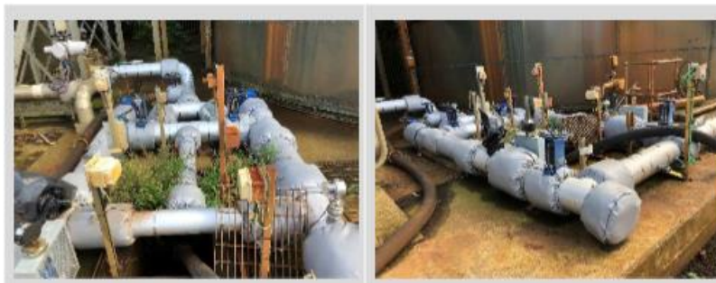
Photos of newly refurbished pipework configuration at unthickened sludge tanks
