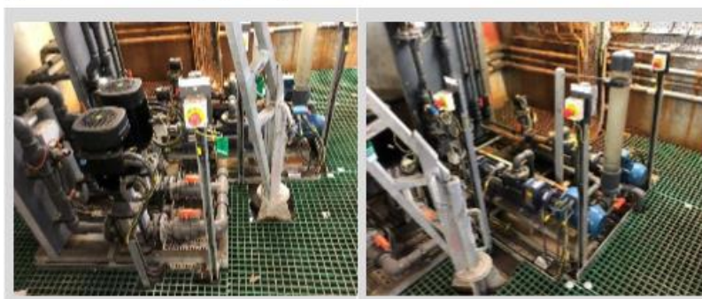
Photos of polymer dosing equipment in bunded area
