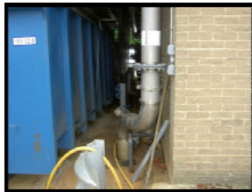
Photo showing liquor pipework leaving the building entering the drainage system
