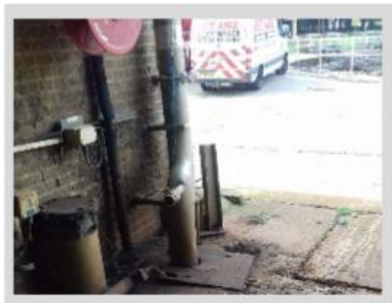
Item no. 12 on drawing no. SK-N001. The pipework drains the liquors from the centrifuge to the external drainage system at point D. The pipe is a below ground non-pressure pipeline and was therefore inspected by means of a CCTV survey. The pipe passed this inspection as no Grade 3, 4 or 5 defects were recorded (no defects of any grade were recorded). A copy of the CCTV survey report can be found in appendix C (See survey section 7).
