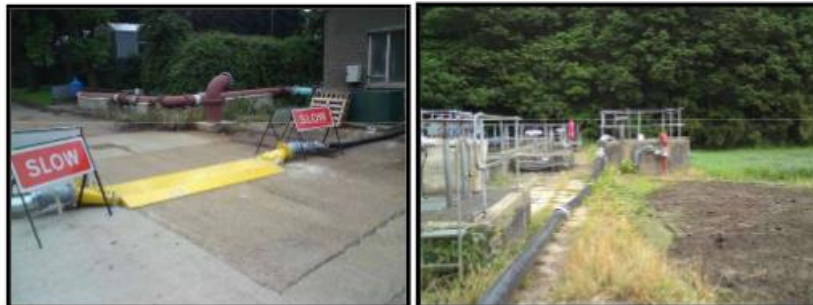
Photos showing replacement above ground pipework for the liquor rising main
