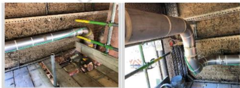
Photos of above ground unthickened sludge pipework to centrifuges with lagging removed
