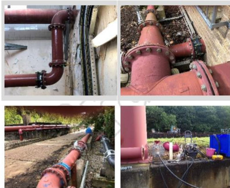
Photos of above ground sections of liquor return pipe including pressure test equipment for below ground sections (bottom right)
