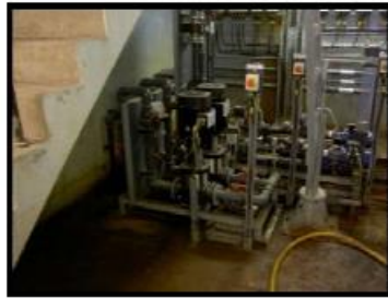
Photos showing new polymer dosing equipment
