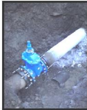
Photo showing new valve installation at the upstream end of the rising main
