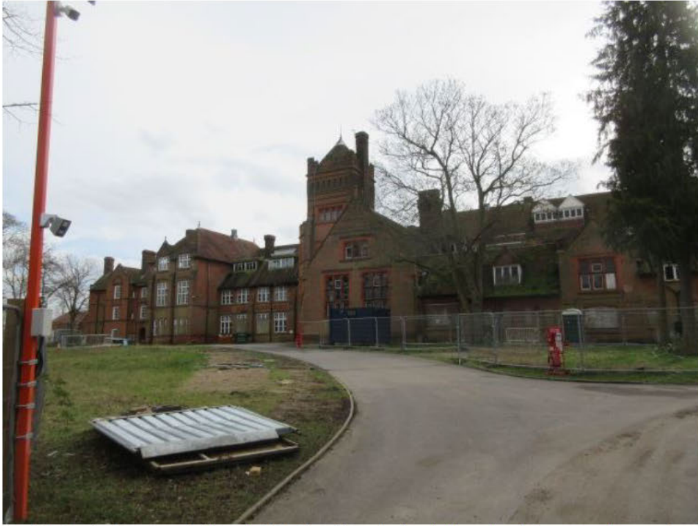
Plate 1: Former Friends' School main building, looking south east
