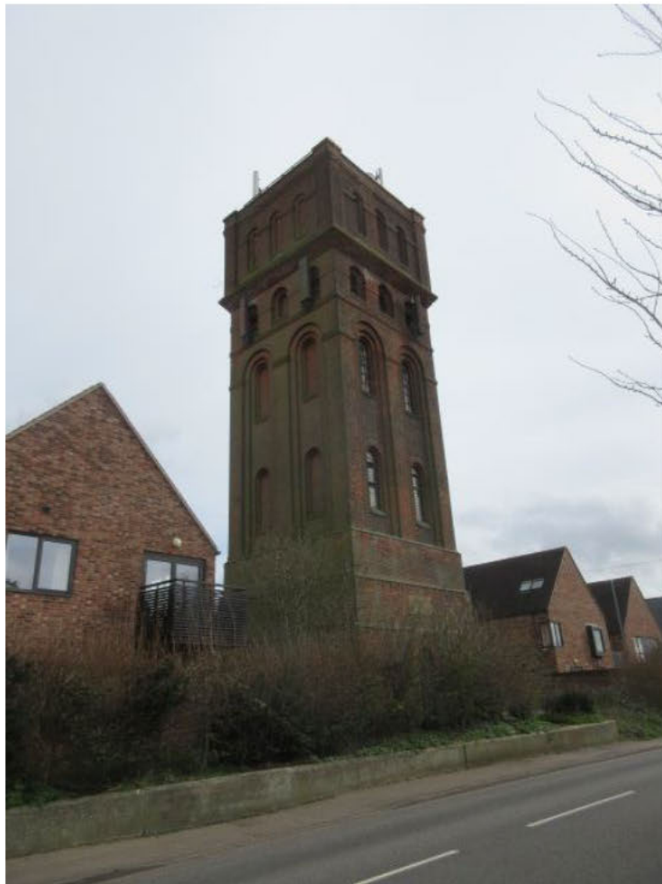
Plate 4: Listed water tower, looking south east
