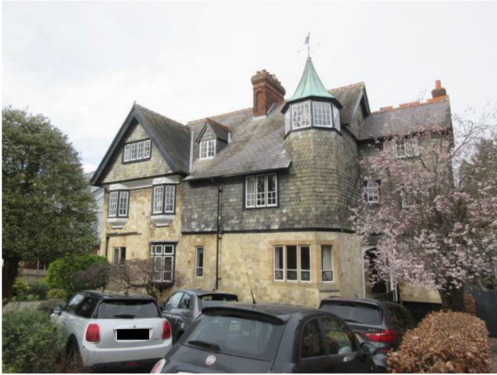
Plate 3: Nos. 9 – 10 Mount Pleasant Road, looking north west
