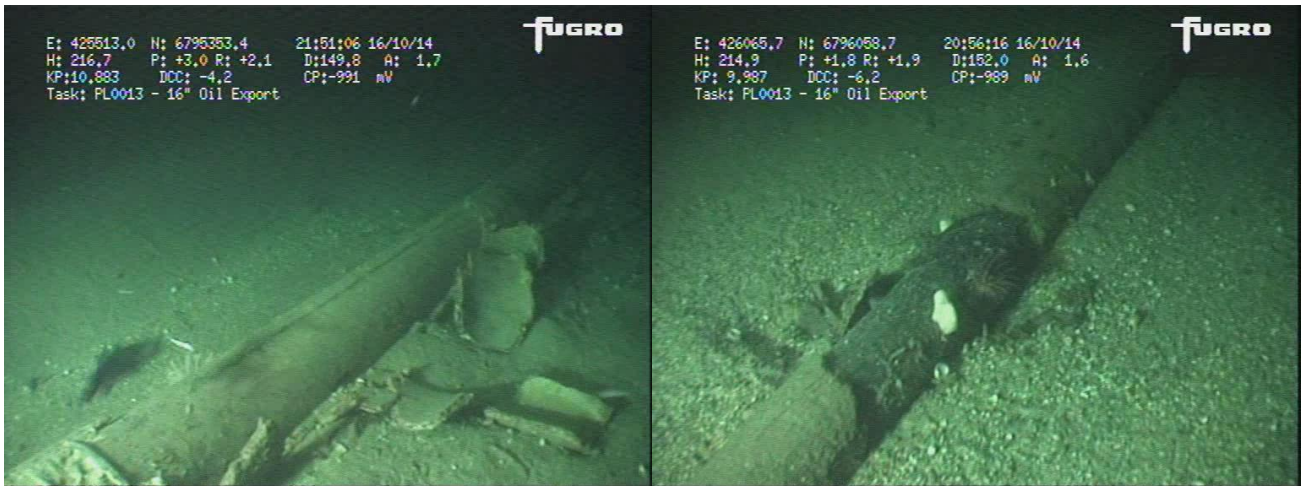
Figure 4.2.1: PL13 examples of degraded CWC (2014)
