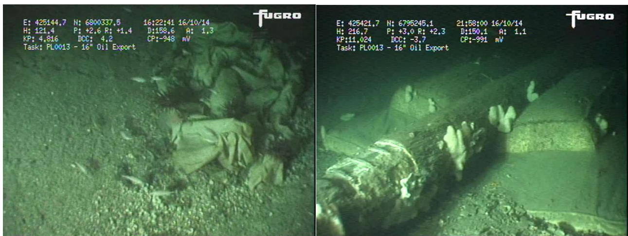
Figure 3.5.1: Examples of grout mattresses used for remediation (2014)
