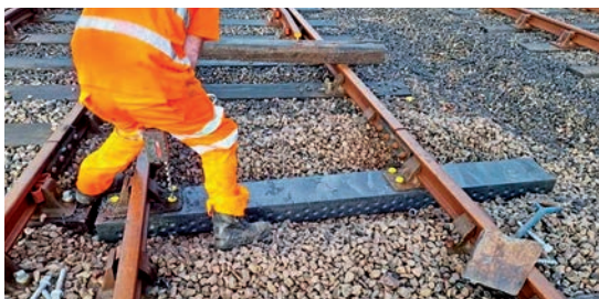
NTS carrying out installation of the composite sleepers.
