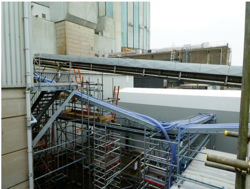
Photograph 17: Vacuum Fill House Exterior with pipework to transport wet waste
