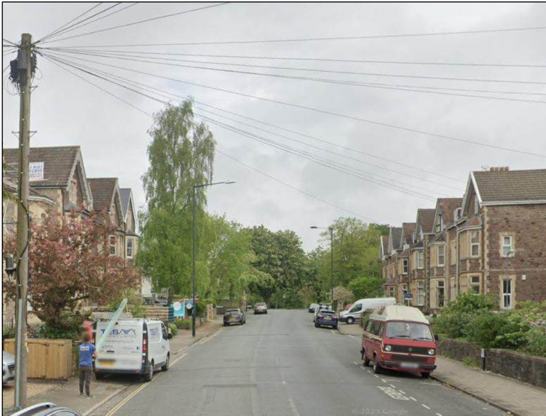
Photograph 4 – Redland Road (looking north)
