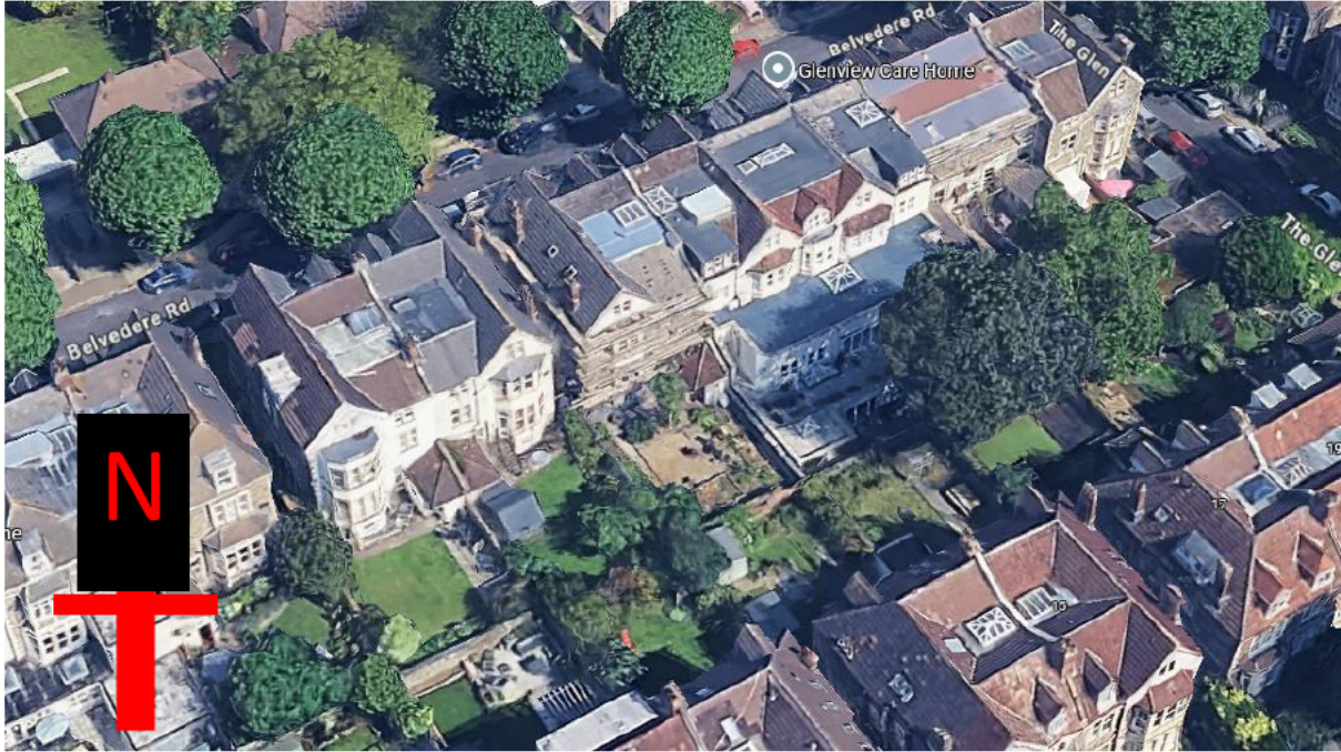
Fig. 1 – Aerial Image of the Site – Overshading Risk
