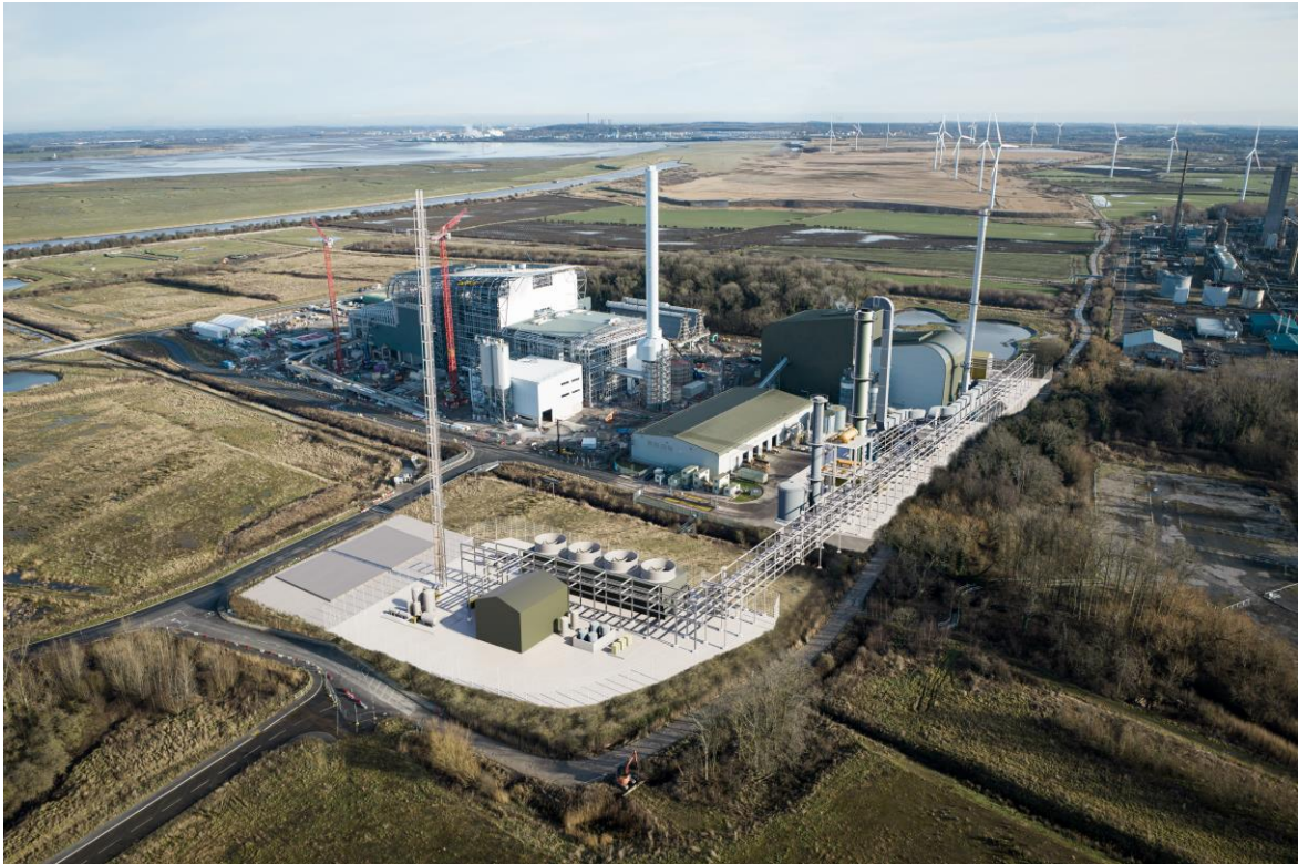
Image: Protos Energy Recovery Facility with Carbon Capture – image shows the Encyclis ERF under construction (left of picture) which was recently permitted for CCS and the operational Evero Energy biomass ERF (right of picture) with proposed CCS plant in foreground.
