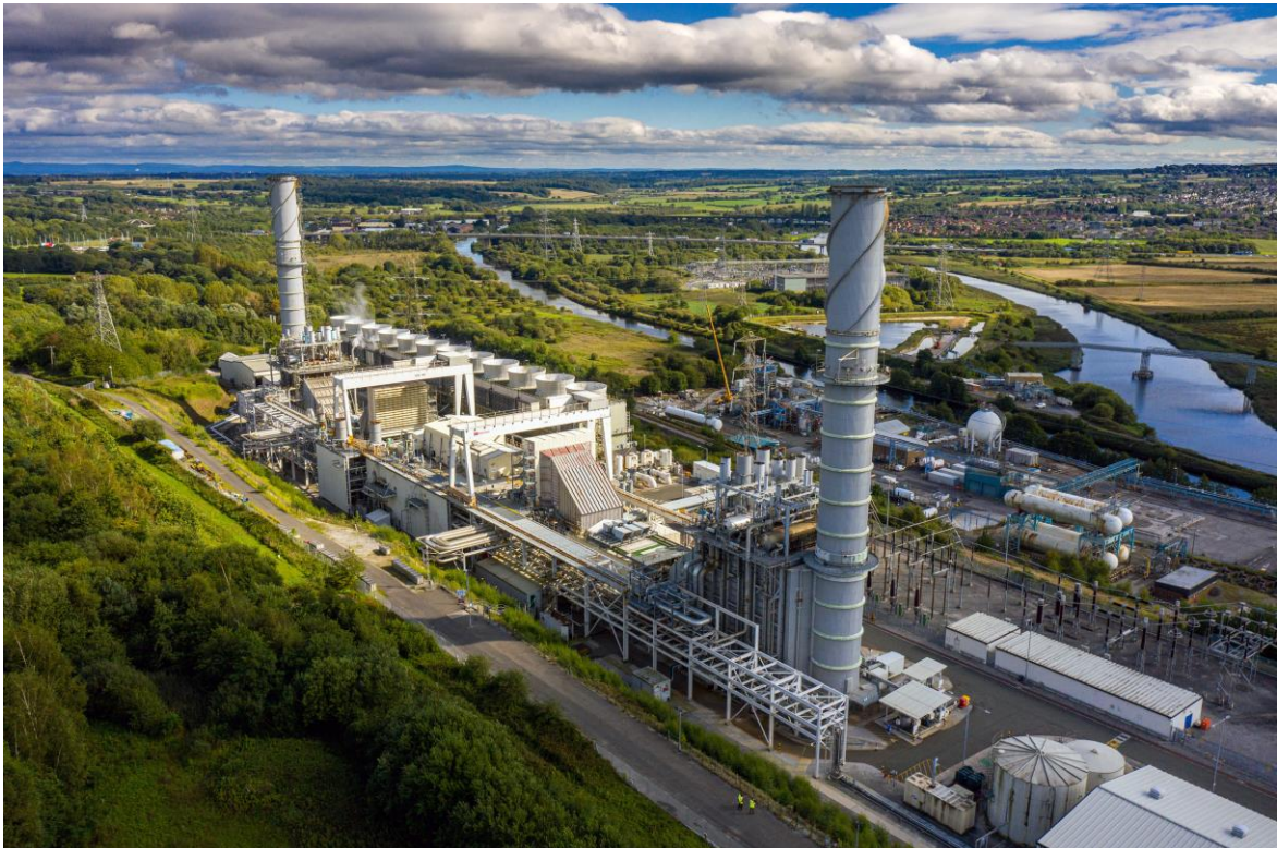
Image: Intergen CCGT Power Plant, Runcorn with a view over Cheshire in the background. Intergen will be supplied with blue hydrogen from HyNet main and will operate on a mix of natural gas/hydrogen. Image supplied by Progressive Energy.
