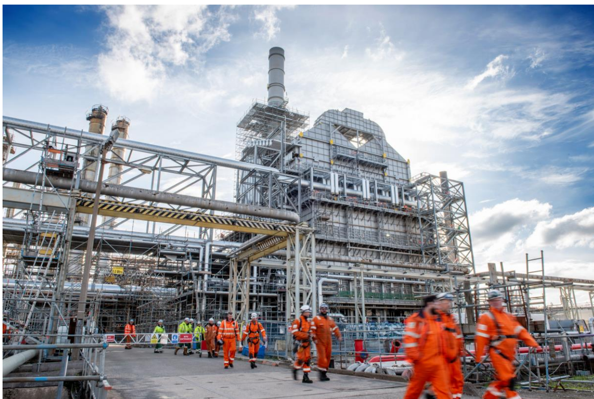
Image: Stanlow Refinery in Ellesmere Port. Image supplied for use by Essar Energy. – Image is of the new furnace, which is the first of its kind in the UK, capable of running on a 100% hydrogen source and will replace three existing furnaces at Stanlow. It is helping to reduce CO 2 emissions by more than 240,000 tonnes each year from 2027.
