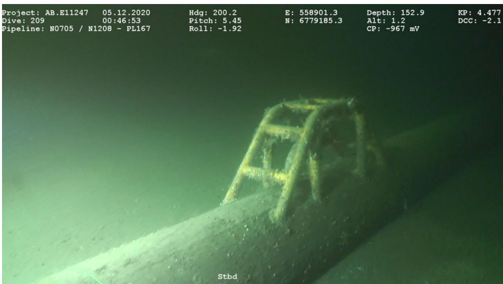
Figure 15-2 Vent valve (example)
