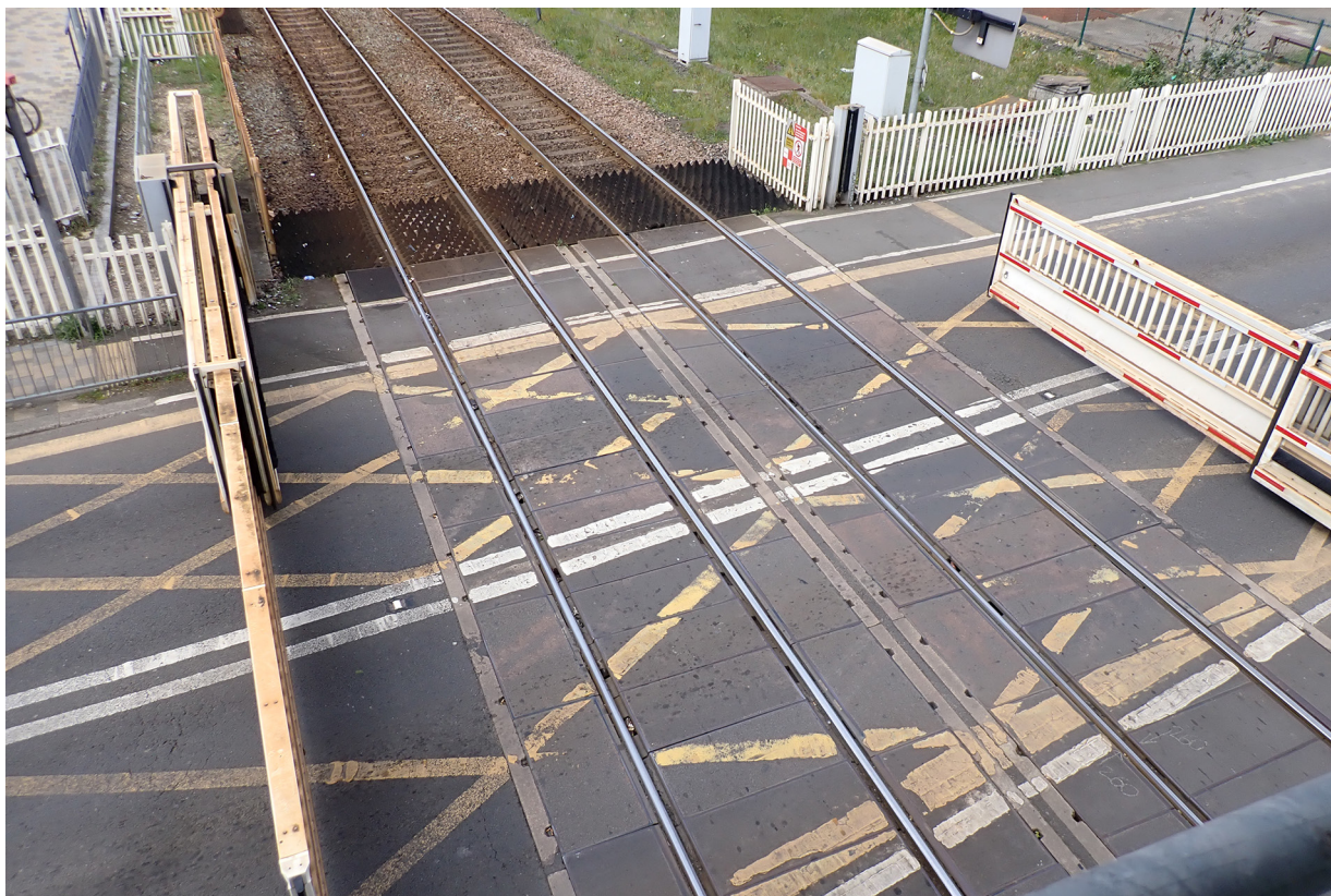
Figure 12: View of Redcar level crossing from the operator's pedestal.
