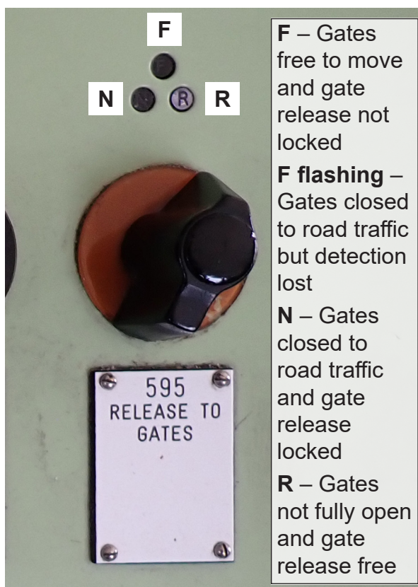
Figure 11: Crossing release indications.
