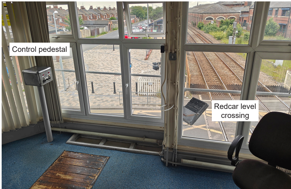
Figure 6: Redcar level crossing and control pedestal.
