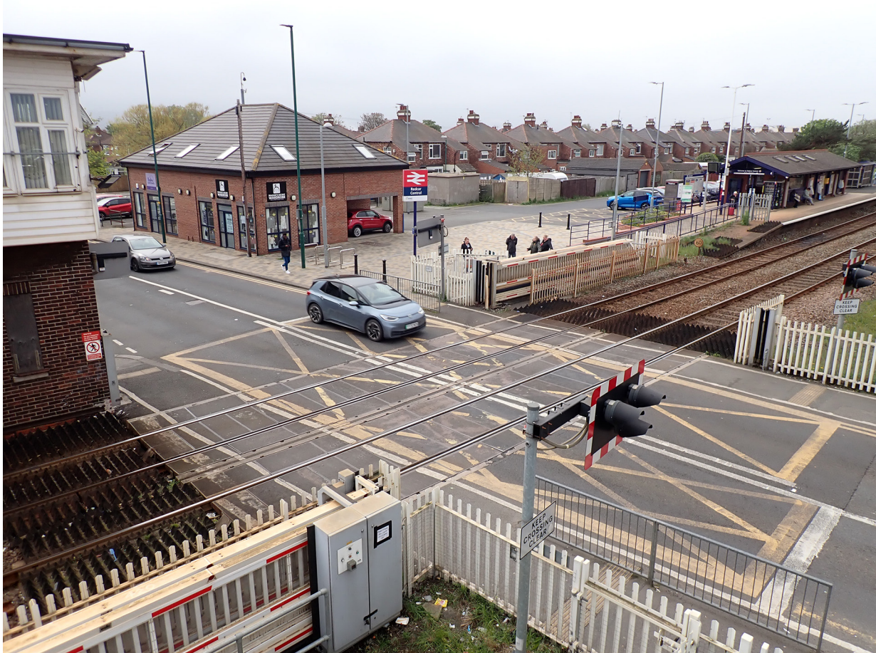
Figure 13: View of Redcar level crossing with the gates open to road traffic.
