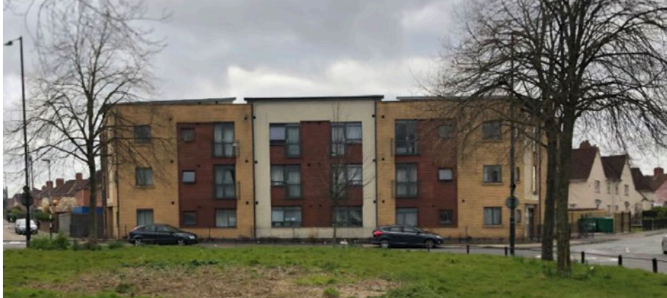
Carpenters Place - Facade
