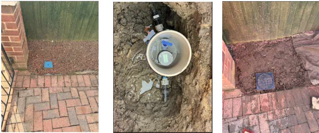
Figure 23: Typical meter replacement (Before, Remove, Replace)
