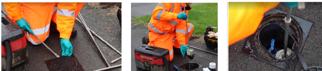
Figure 23: Typical meter replacement (Before, Remove, Replace)
