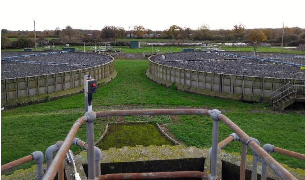
Figure A12-6 – Secondary biological treatment (Process type – trickling filters) at Wincanton WRC.
