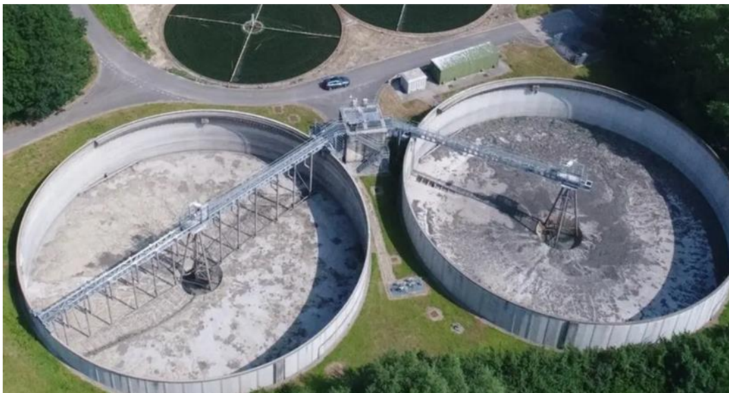
Figure A12-3 – Storm tanks at Saltford WRC.
