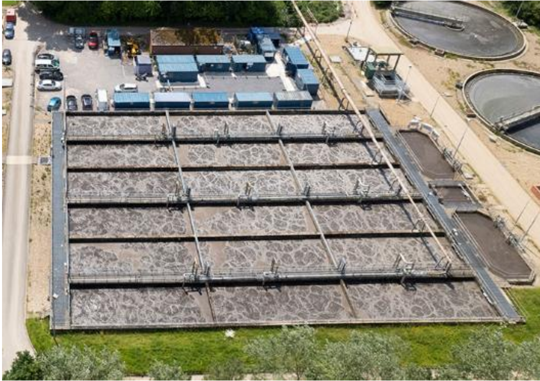
Figure A12-5 – Secondary biological treatment (Process type - activated sludge plant) at Holdenhurst WRC.
