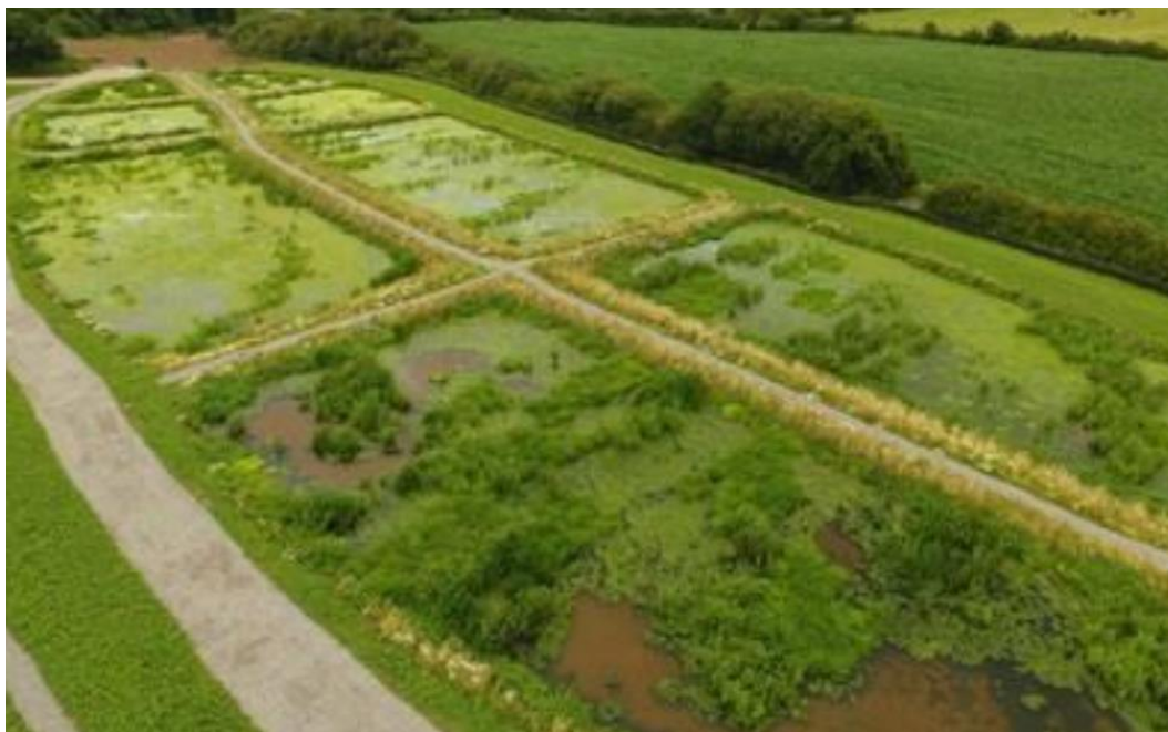
Figure A12-7 – Cromhall Integrated Constructed Wetlands used to treat sewage effluent.
