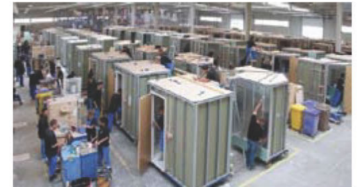
Off-site construction for bathroom and kitchens is more likely in a tall building. Ensure lifts and corridors are wide enough to enable new pods to be installed over time without too much disruption
