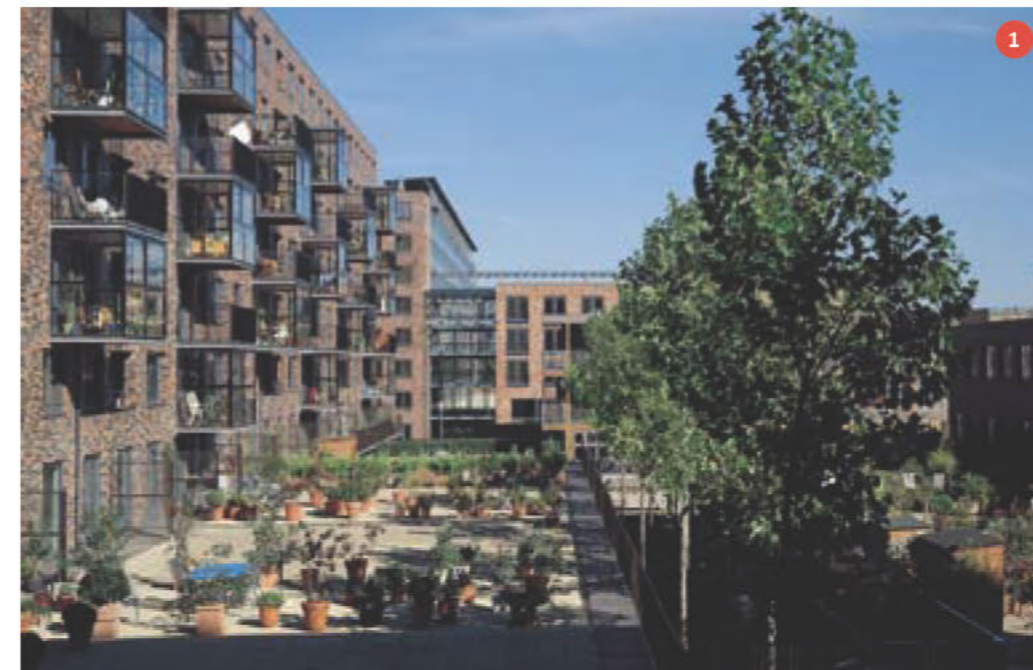
1 Apartment block providing a range of communal and private outdoor spaces (balconies, wintergardens, and courtyard space above a parking podium). Trees are allowed to grow up through a slot in the podium. Architect: KCAP Architects&Planners, Photo: a+t / César San Millán
