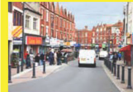
1 East Street, Bedminster (uniform prevailing building height)
