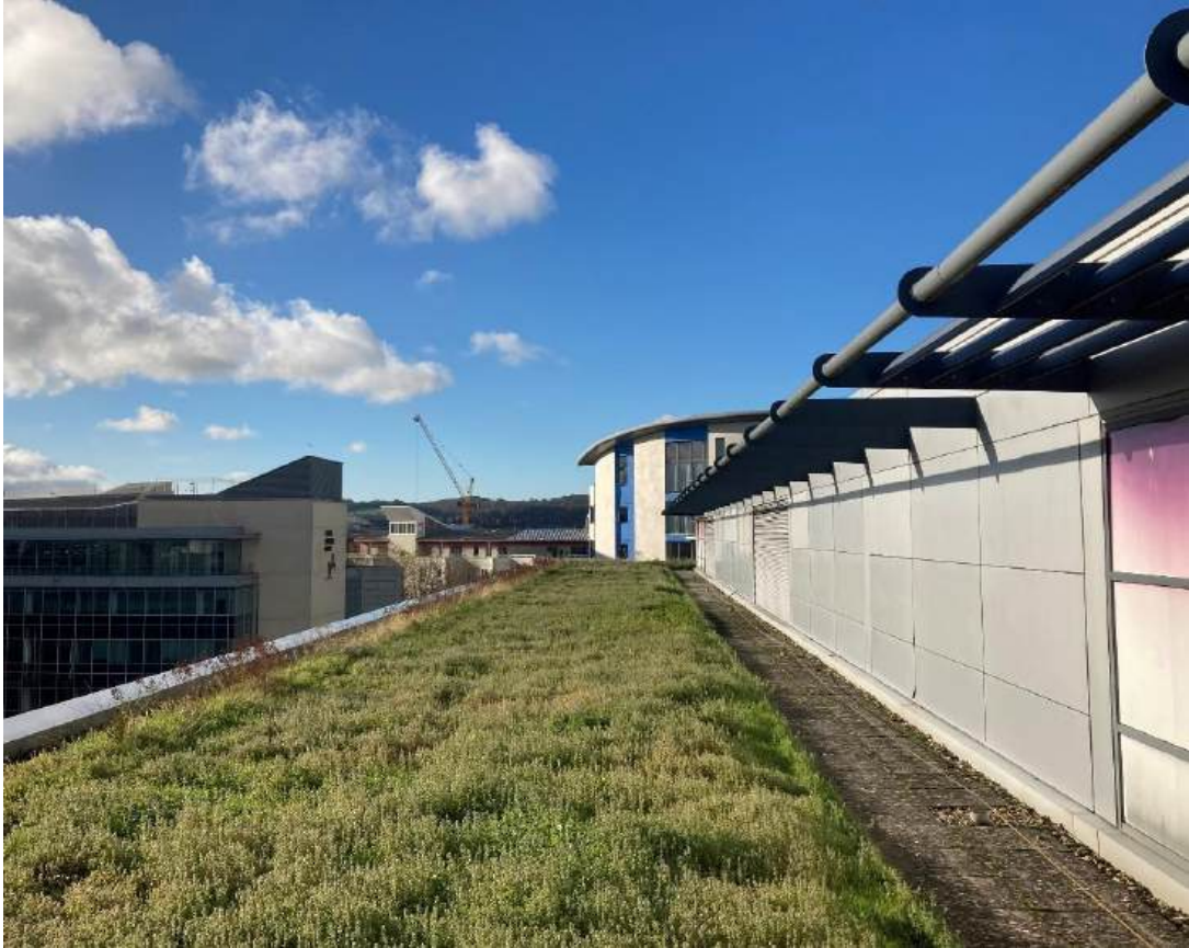
Image 7 – Existing Means of Escape
