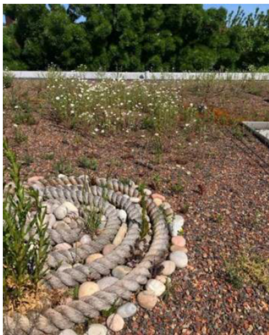
Plate 1.5 Rope coil on biodiverse roof
