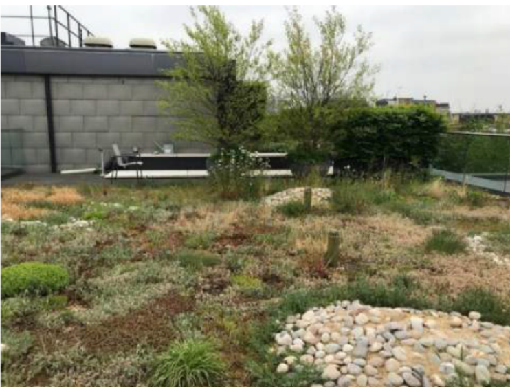
Plate 1.4 Sandy piles on biodiverse roof
