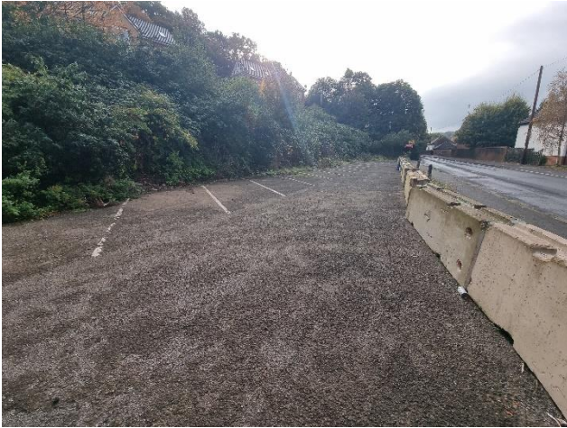
Photograph 7. Hard-standing to the south of the building.
