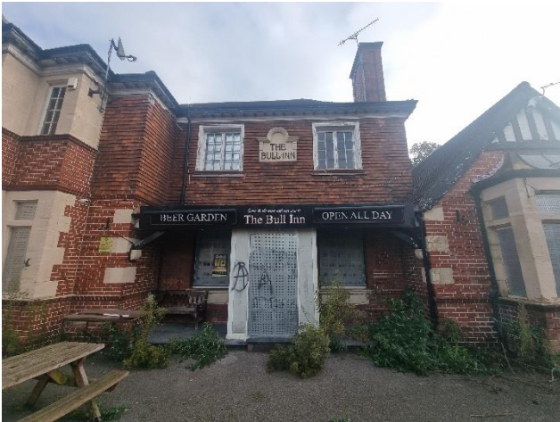
Photograph 1. The Bull Inn viewed from the west.
