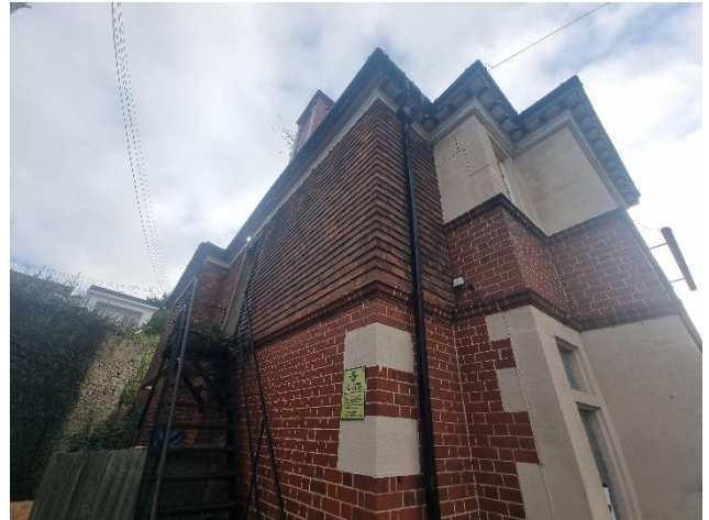
Photograph 2. Detail of the north-western corner of the former pub building.
