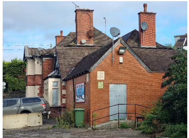
Photograph 4. General view of the former pub building from the south.
