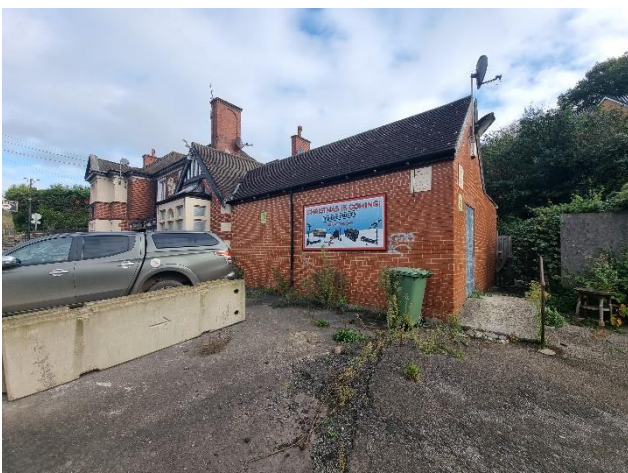
Photograph 5. General view of the building from the south-west.
