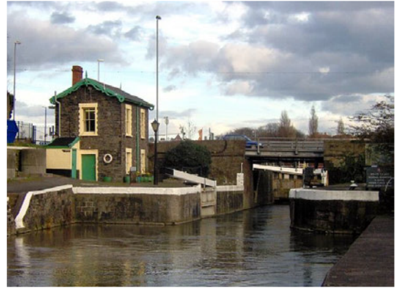
Netham Lock and Bridge
