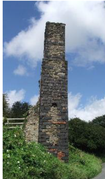
Chimney: Former lower engine house.
