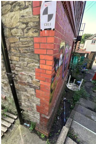
North brick & east stone wall
