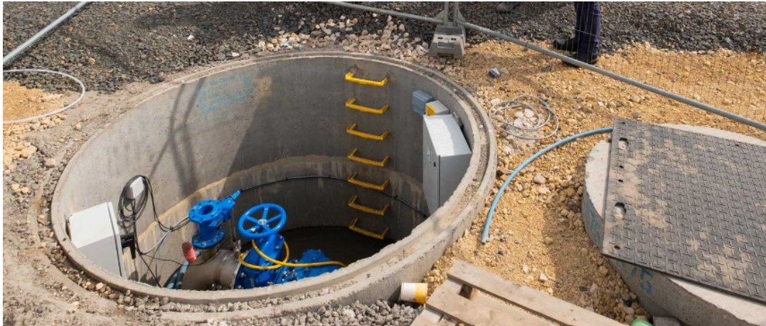
Figure 17: Borehole used to abstract mine water for Gateshead district heating scheme. Source: Coal Authority, 2023
