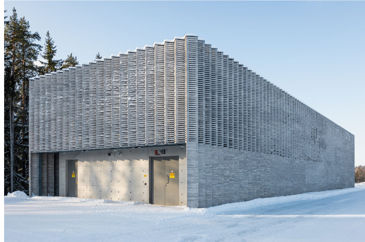
Project: Imatra Electricity Substation, Imatra, Finland Architect: Kivinen Rusanen Architects Client: Fingrid Photography: Tuomas Kivinen
