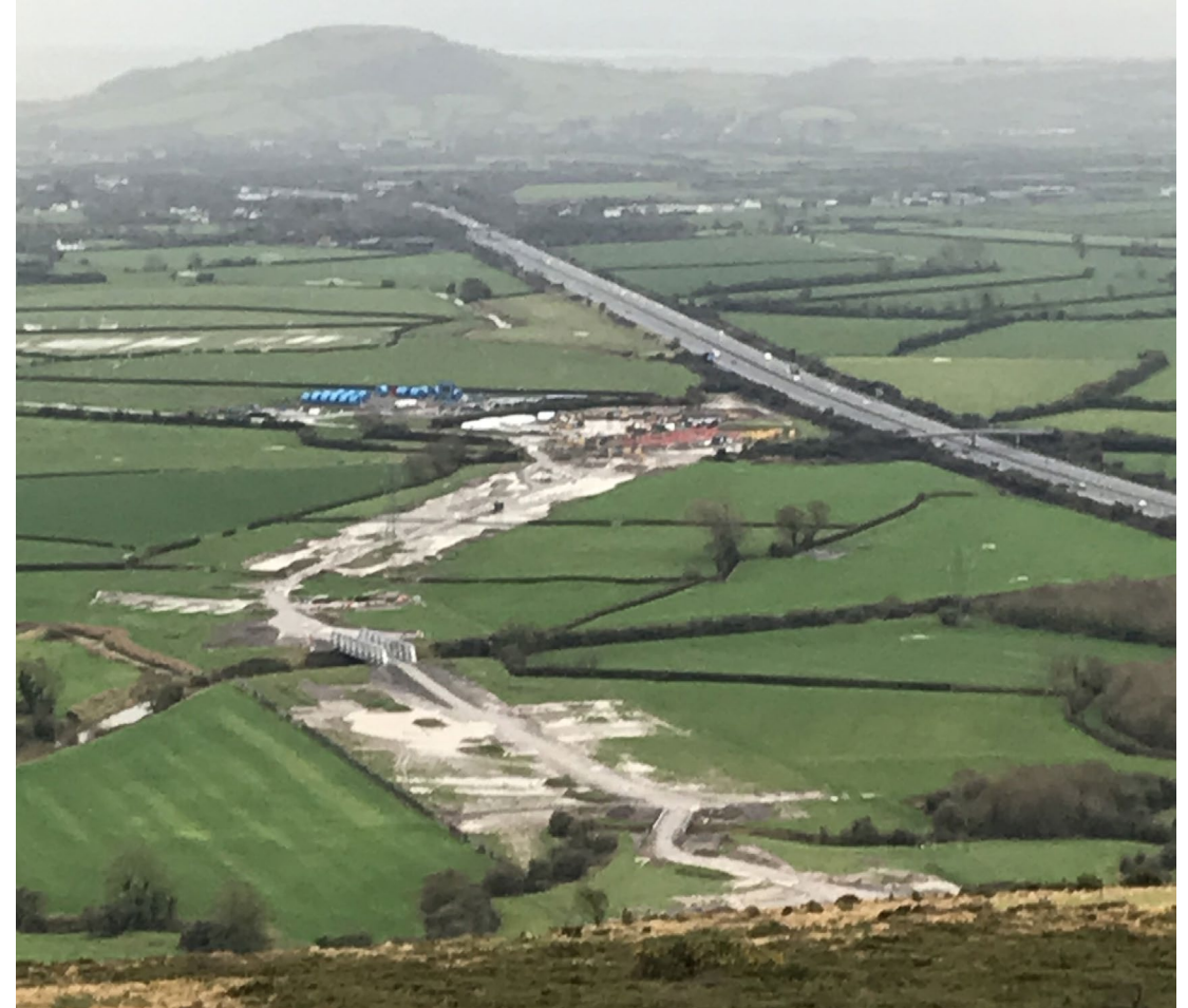
Cable sealing end compound works area for HPCC from Crook Peak
