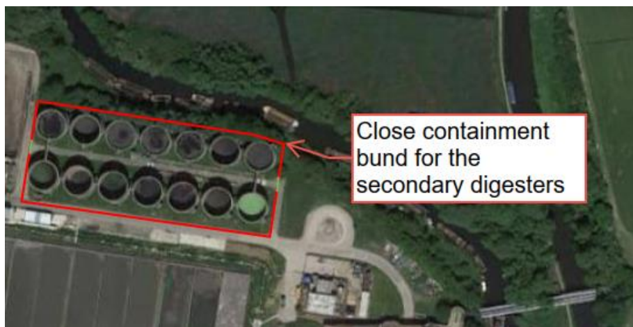
Figure 4-4 – Close Containment Bund for the Secondary Digesters
