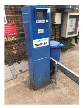
Sludge reception tank and import logger. Imported sludge is discharged into this reception tank, which is screened and passed to the blending tank.
