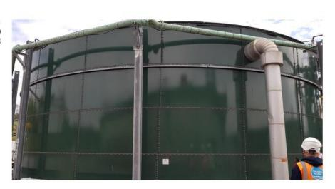
Photo of one of the eight primary digester tanks on site. Digested sludge is transferred to the secondary digester tanks.
