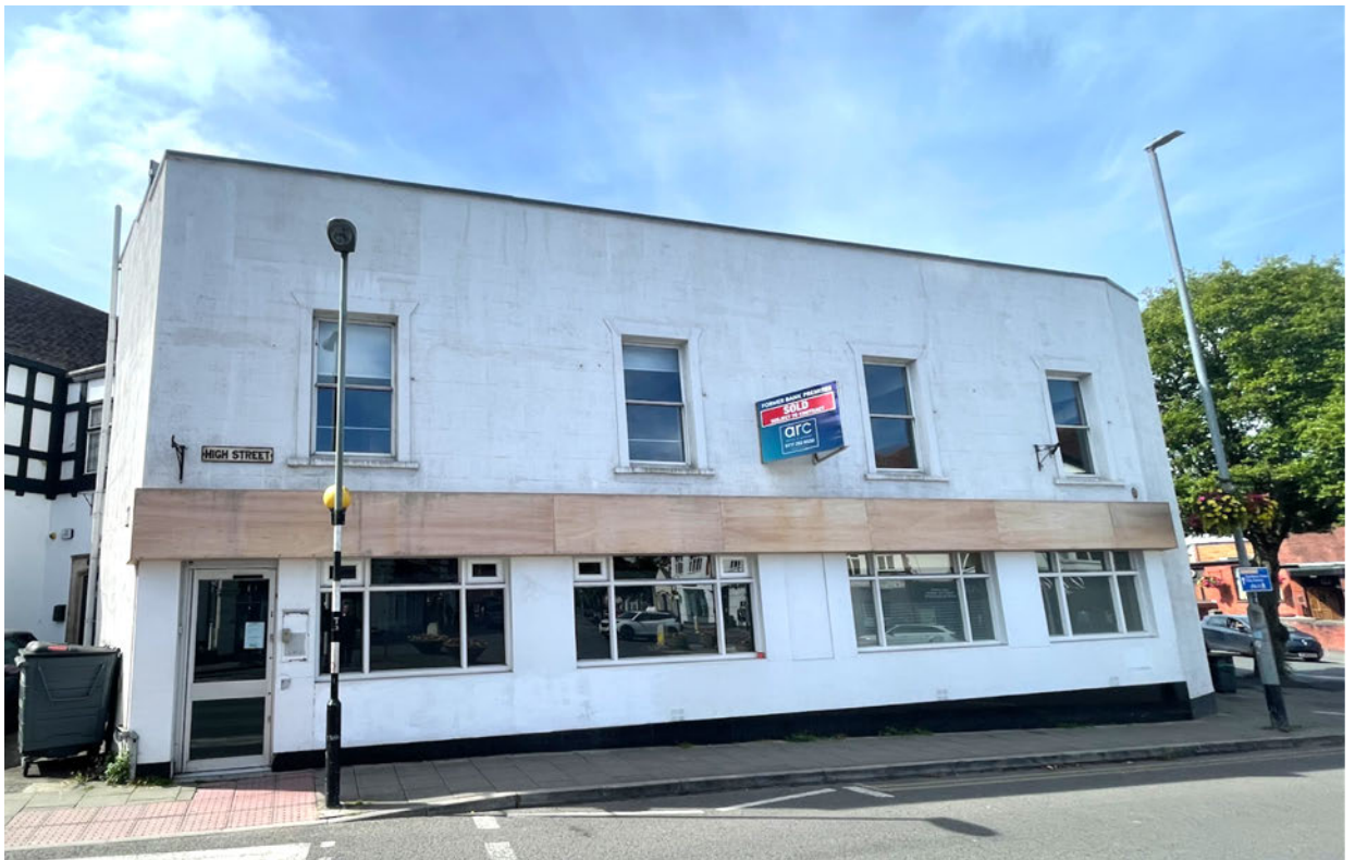
Image of the existing former bank building viewed from the road
