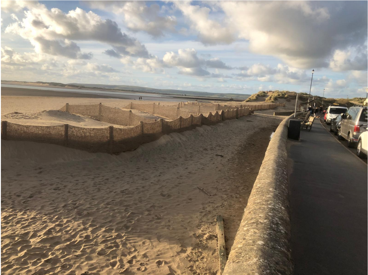
Figure 35 - Sand dune restoration in Instow, Devon (image credit: Sophia Craddock, Environment Agency)
