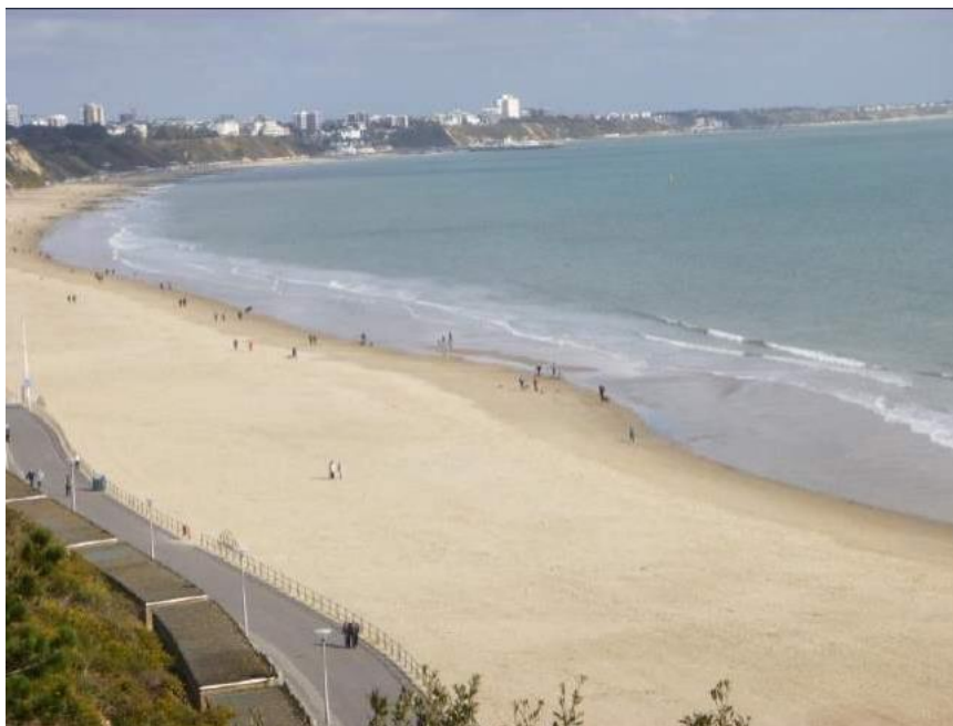
Figure 33 - Beach nourishment at Poole Bay. Image credit: Dave Robson, Borough of Poole
