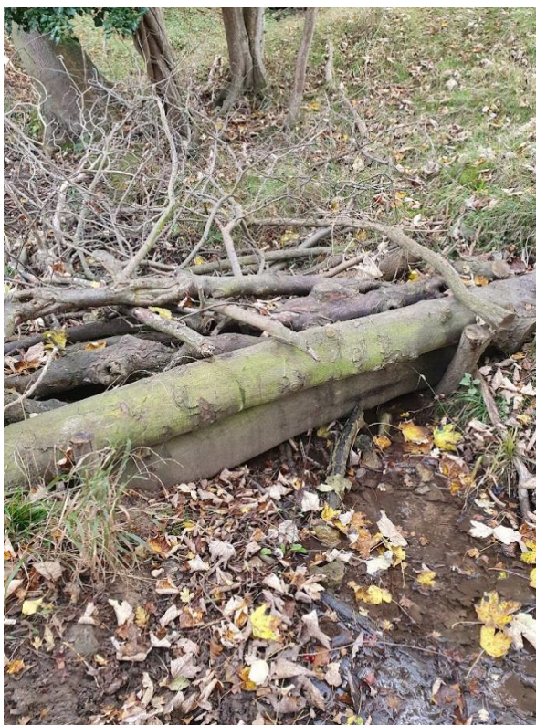
Figure 11 - An example of a leaky barrier in the Cotswolds (image credit: Jenny Broomby, JBA Consulting)
