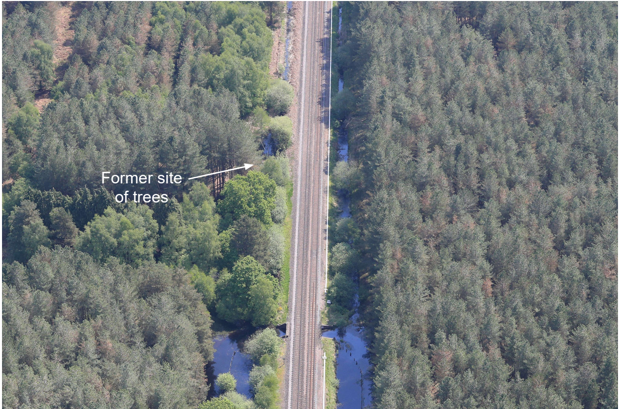
Figure 7: The extent of flooding at the site in May 2024, just over 3 months after the accident. The previous location of the pine and oak trees is indicated (courtesy of Network Rail, with RAIB annotations).
