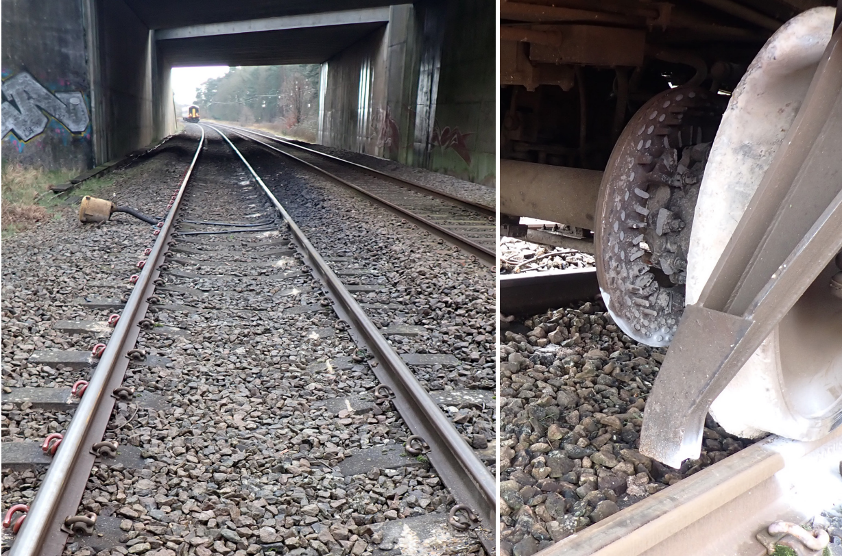
Figure 9: The train's final stopping position beyond the A11 bridge and the sleeper marks made during the derailment (left) and the remains of the axle-mounted brake disc following the train being rerailed (right).
