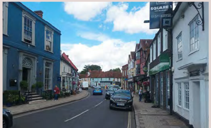
▲ Strong continuous built form frontage reinforces hierarchy of character and use along High Street, Great Dunmow.
