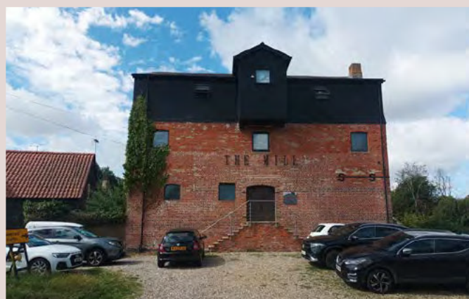
▲ Red brick mill with a retained historic facade converted into non-residential uses in Hatfield Heath
