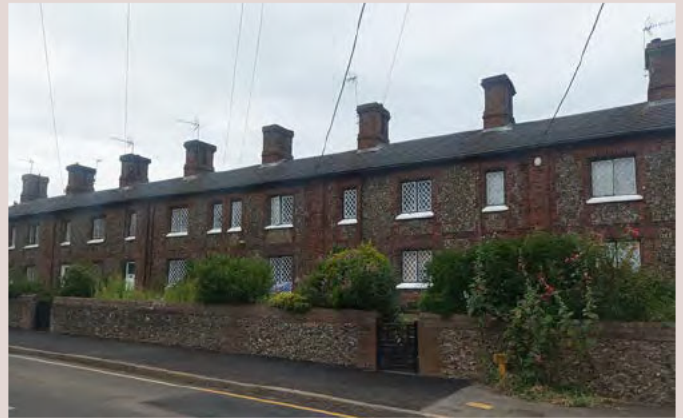
▲ Mid 19th century terraces of flint-faced dwellings create distinctive village character in Wendens Ambo.
