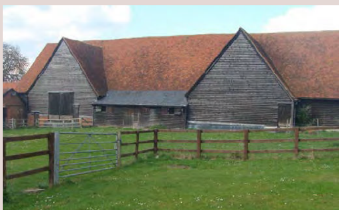
▲ Grade II listed Bury Farm Barn, Felsted, with a restored weatherboarded timber framed and Queen post roof structure.
