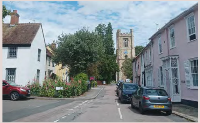
▲ Built form along Church Street retains key views towards St Marys Church.
