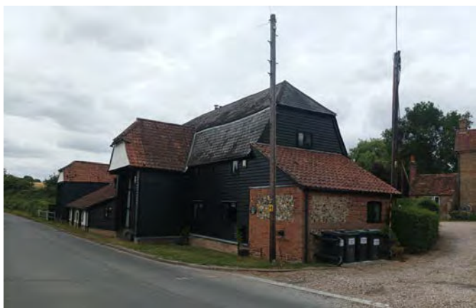
▲ Farmsteads and barns with weatherboarding and flint walls are a common sight within the hamlets of Uttlesford.
