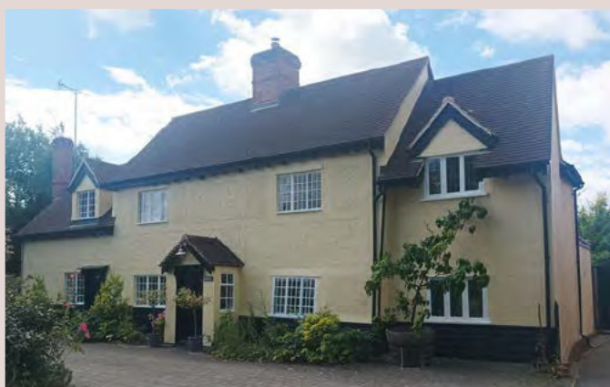
▲ Peg tiled roof, pargetting, dormer windows, central chimney and black weatherboarding on Dunmow Road, Takeley.
