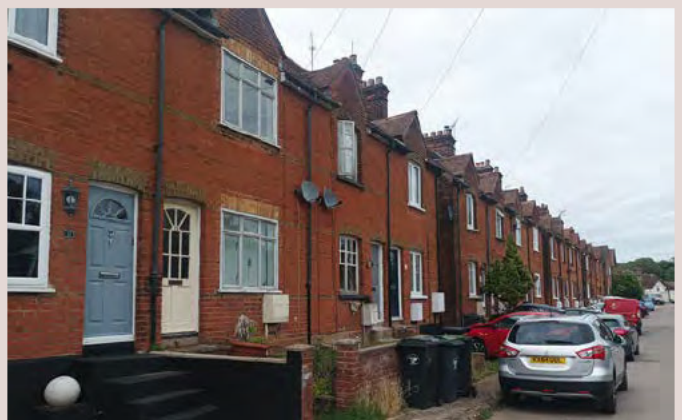
▲ Red brick victoria terraces with raised entrances along Sunnyside create a coherent narrative.
