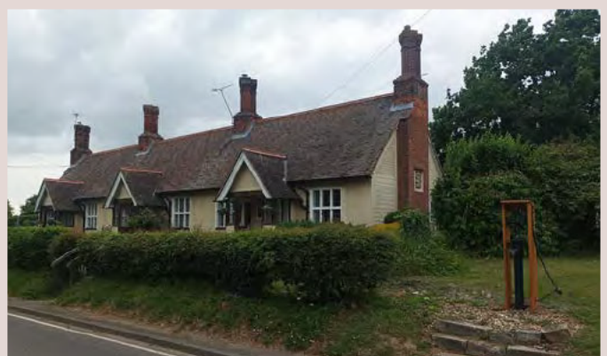
▲ Almshouses in Radwinter - Three gabled porches project on the front. Roofs tiled, with 4 chimney stacks each and casement windows.
