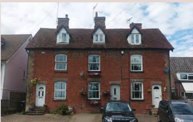
▲ Dormer windows and central stack chimneys create strong character for red brick terraces.
