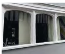
Wooden framed windows
