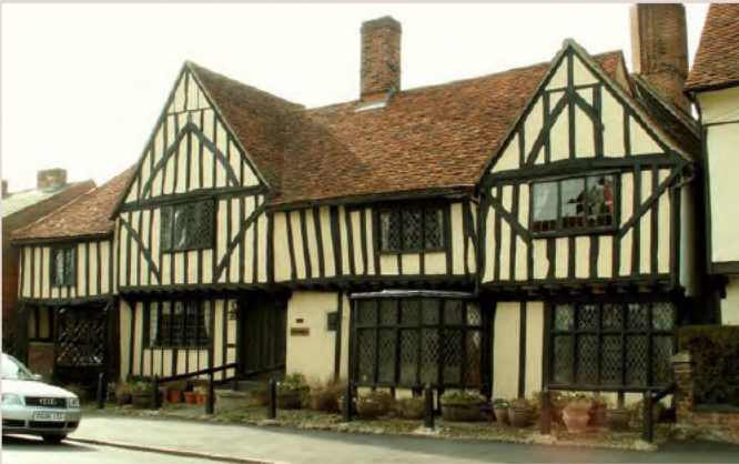
▲ Historic architecture of timber frames and peg tiled roofs on Lower Street.
