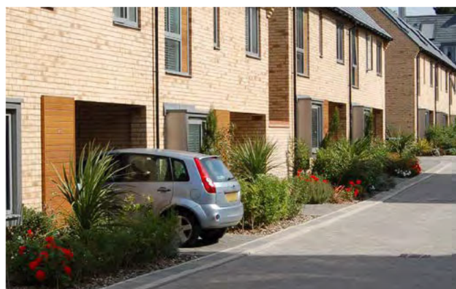
▲ On-plot parking is integrated into the street scene with soft landscaping to create an attractive streetscape.
