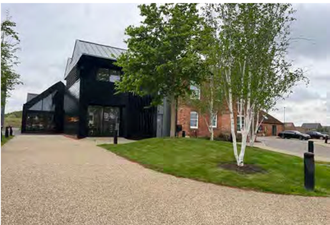
▲ Barn conversion at Houlton, Rugby to provide community uses and a cafe.
