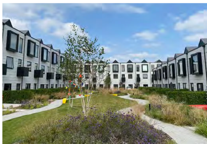
▲ Modular housing provides a resource-efficient method of construction in Port Loop, Birmingham.
