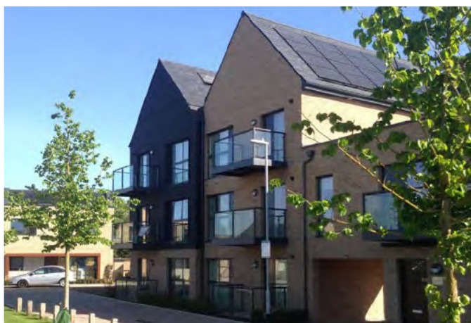
▲ The front and back of the home is clearly defined by landscaping and a front door facing the street. Private balconies are also provided for the homes without gardens.
