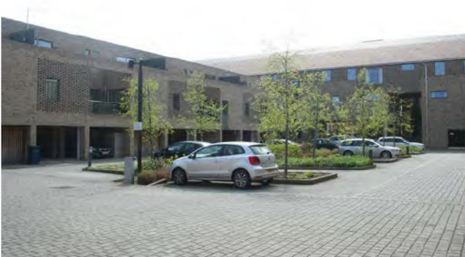
▲ Well-designed parking court with permeable paving and space for servicing and utilities.
