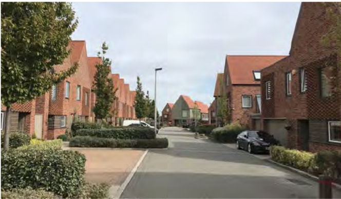
▲ Shared surface streets prioritise safe active travel at Horsted Park, Chatham.
