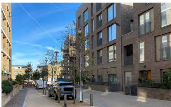
▲ Landscaped and designated on-street parking spaces here in Brentford Locks, discourages anti-social parking.
