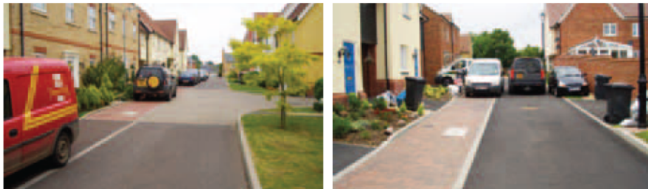
Examples of shared surfaces which are not appropriate for the location, note the indiscriminate parking
