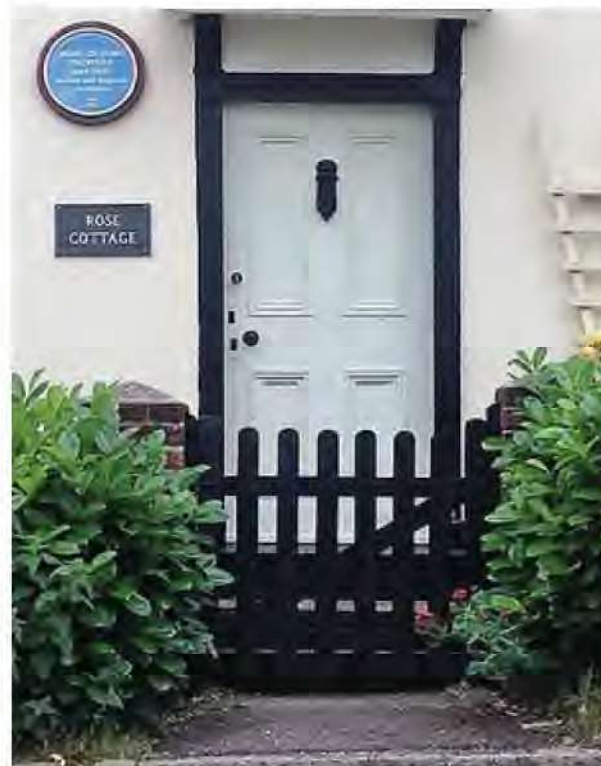
Photo 9. View of House Facade at Church End
