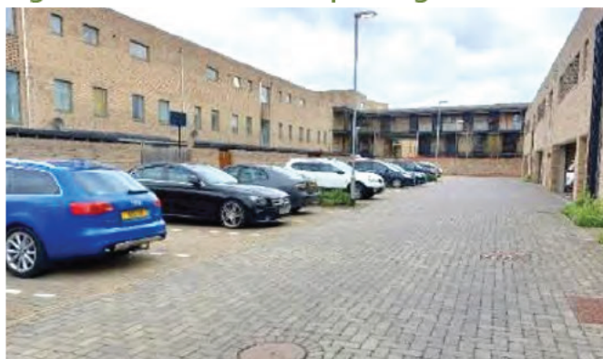
Figure 7-11: Wall-fenced parking courts 43
