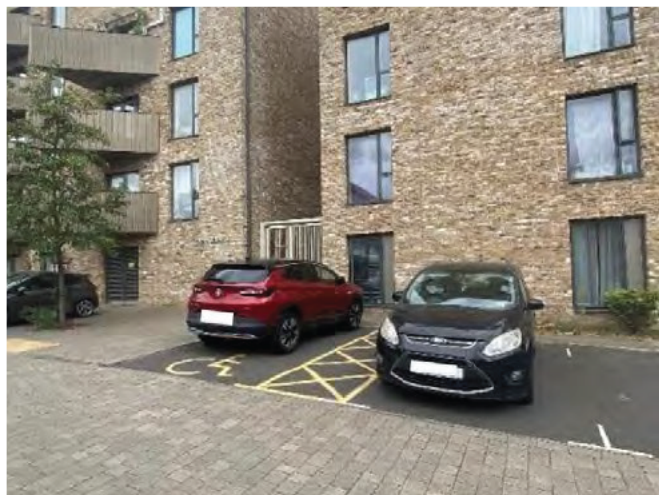
ITP – The Echoes (Grays). Showing a parking space for disabled people in front of a building entrance.
