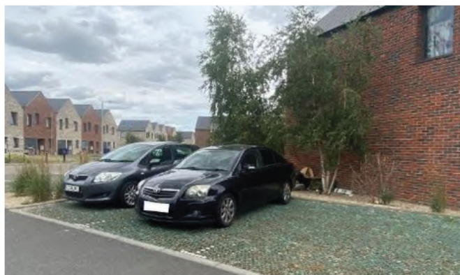
ITP – North View Avenue (Tilbury). Showing grasscrete parking areas, which can be more cost effective to remove compared with traditional surfaces (although maintenance implications of grasscrete should be considered).
