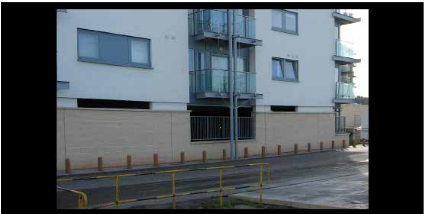
Poorly designed under-croft parking creates dead fronts and divorces the building from activities on the street
