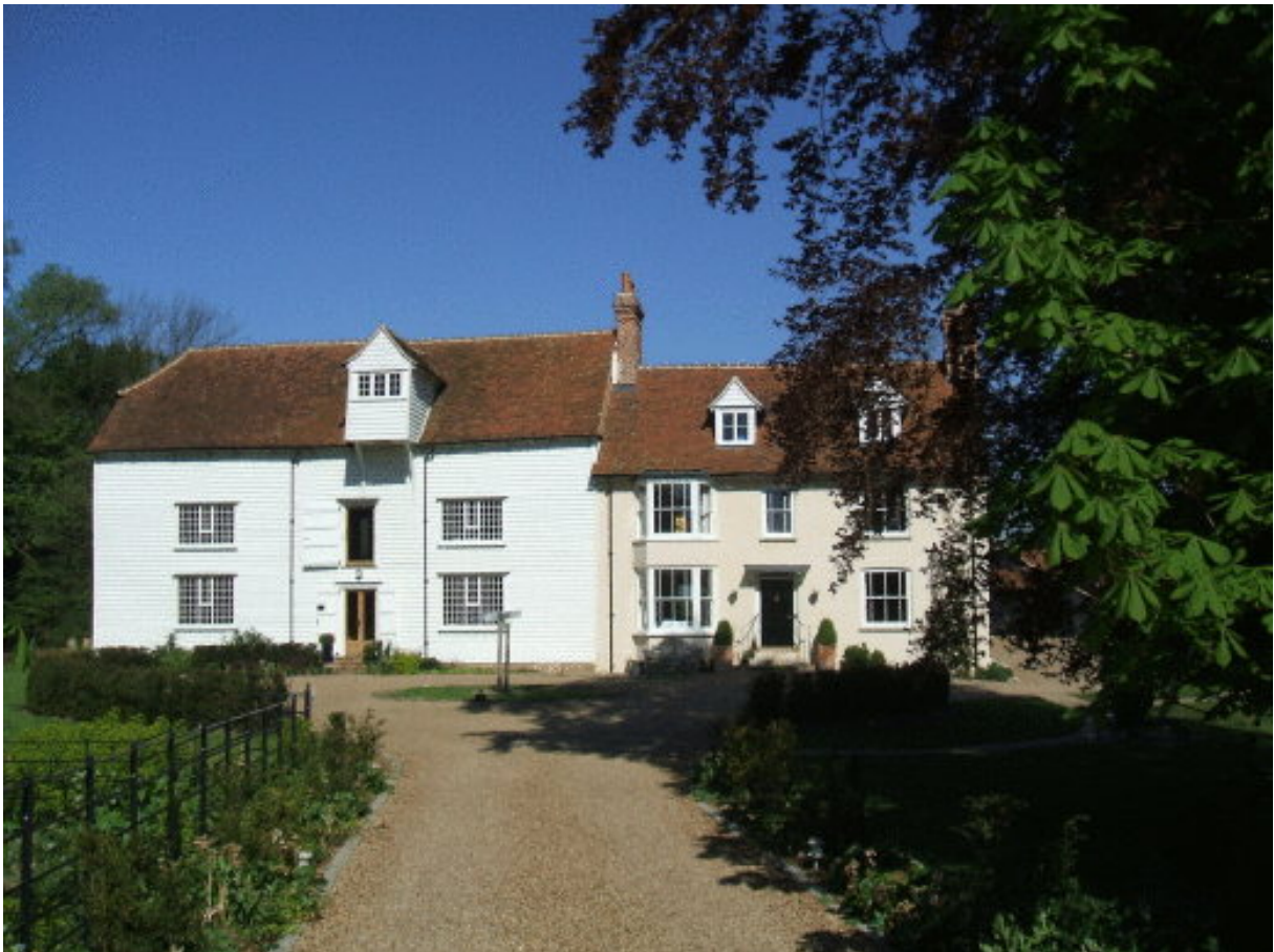
Picture 1.25 Stebbing Mill and Mill House, 18th century important buildings in unspoilt setting
