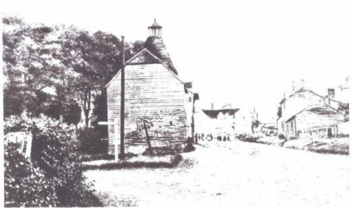
Picture 1.16 Historic View of Church End towards Red Lion with Maltings in foreground
