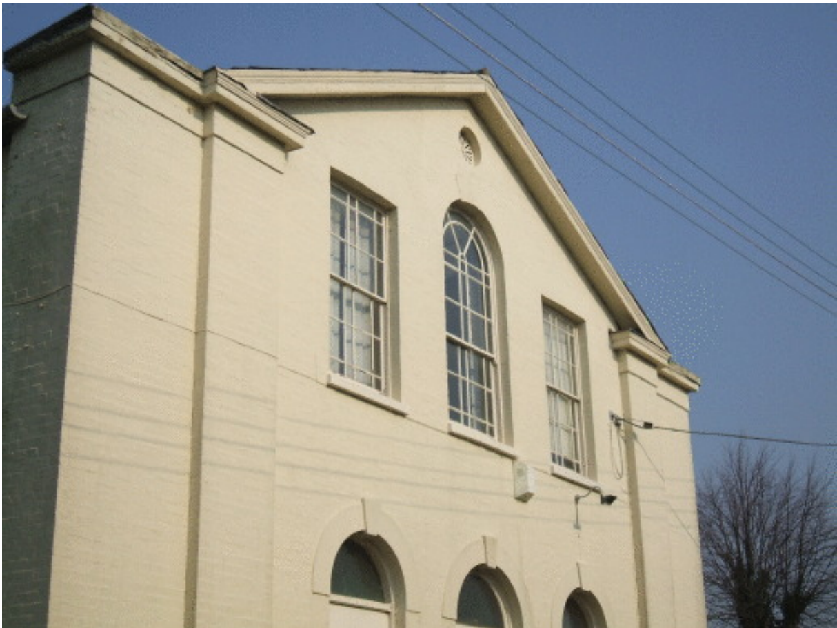
Picture 1.27 Former Methodist Chapel, dominant and important building
