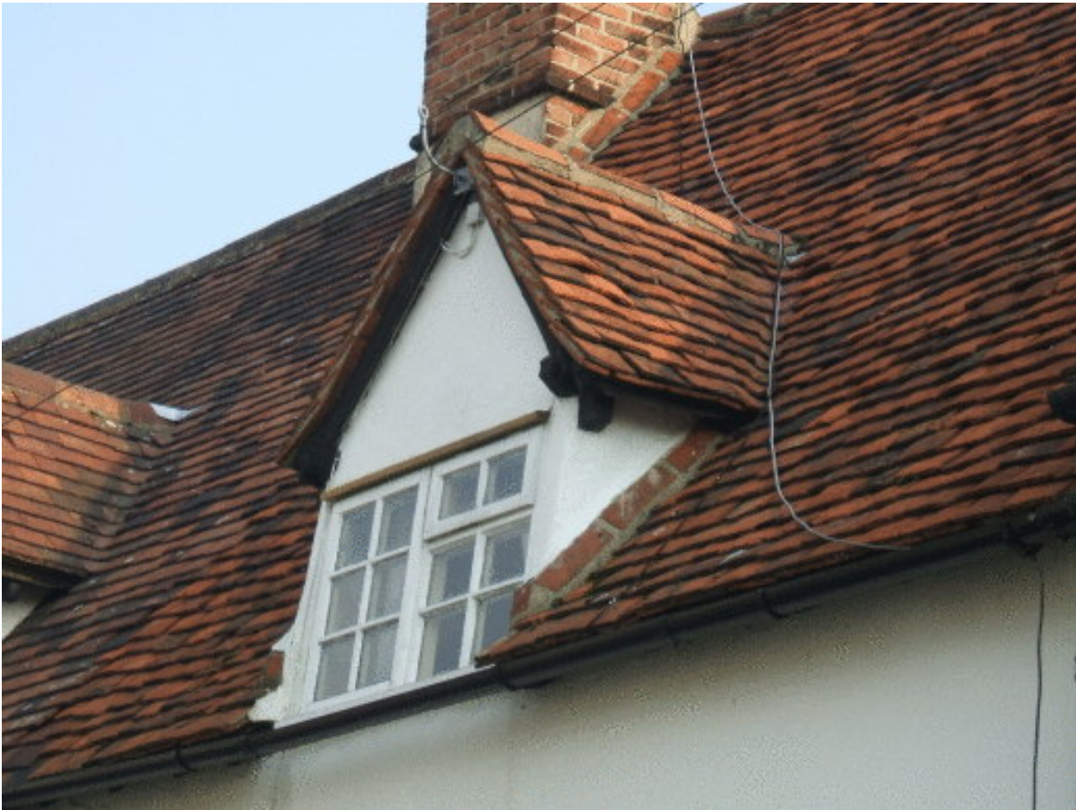
Picture 1.7 Typical small dormer
