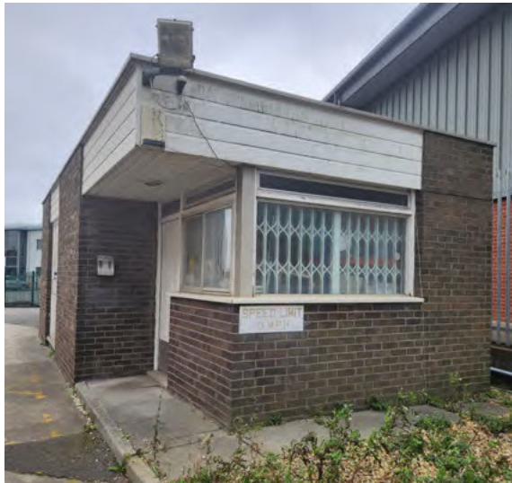
Office portion of substation to be demolished.
